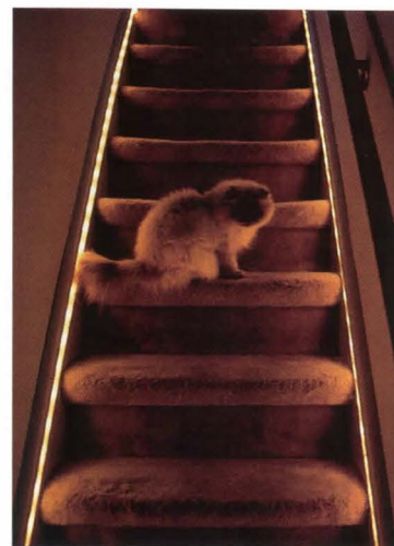
Low-voltage light strips on the stair risers are activated by a concealed motion sensor. The cat is an optional component.
