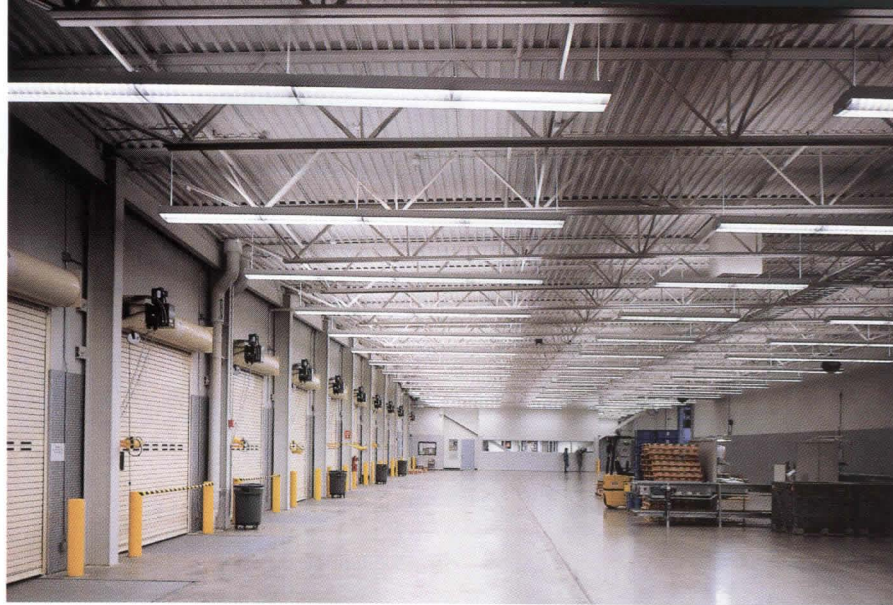
In the warehouse, left, forklift operators moving materials on pallets need to be able to read shelf labels quickly. In the shipping area, above, light from the luminaires reflects off white-painted ceiling, trusses, and walls to produce very uniform illuminances.
