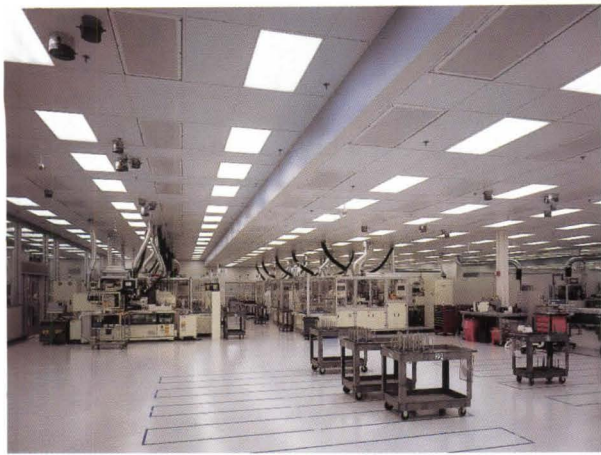
Printing and replication areas (above) needed lighting that met clean-room standards and gave uniform illumination over floor areas. The staging area (right) is a long, narrow room, also with strict clean-room requirements. Here, technicians perform extremely varied, difficult, and critical visual tasks.
