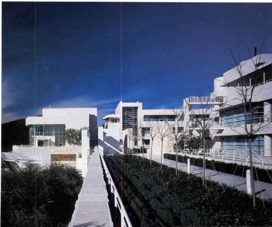
Left: View looking north, with the auditorium (left), the North Building (right), and the East Building (right foreground). The various buildings are connected by walkways and exterior stairs.
