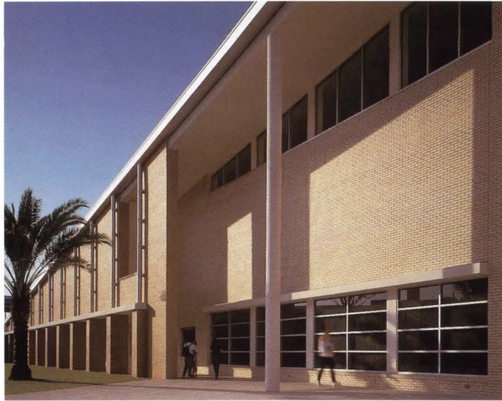
Covered corridors on the classroom building (far left) reduce energy-consuming air-conditioned space. Overhanging eaves on the media center (left) protect the interior (below) from direct sun.
