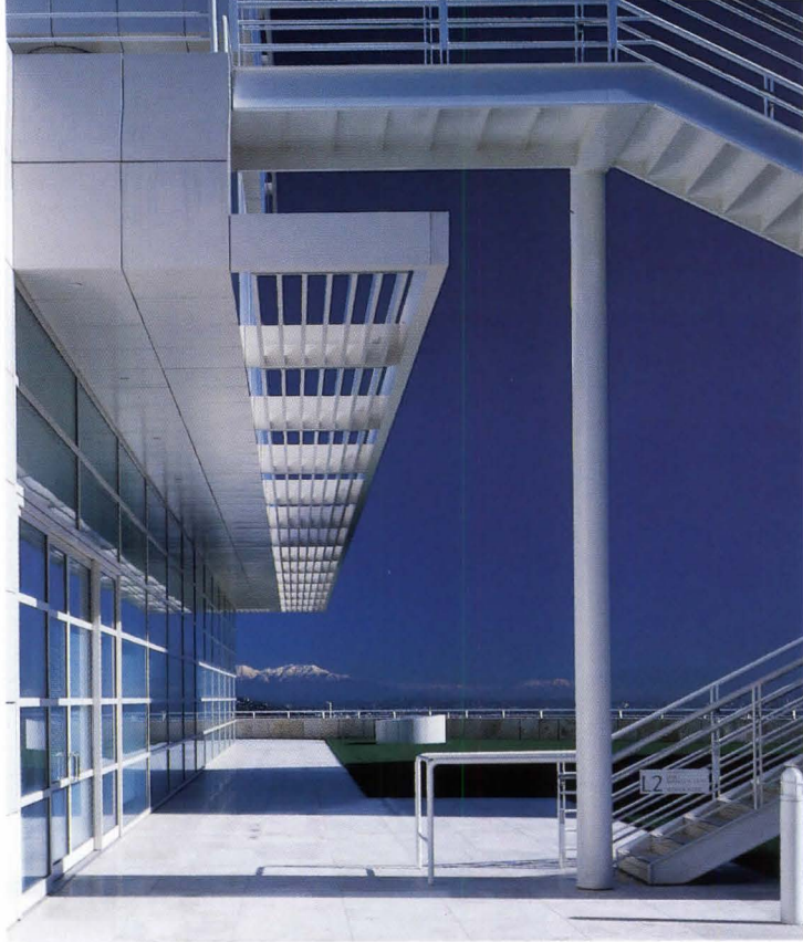
Left: On a clear day, views from the Getty Center reach as far as the snow-capped mountains to the east. Brise-soleils provide much-needed sunshading to the East Building.
