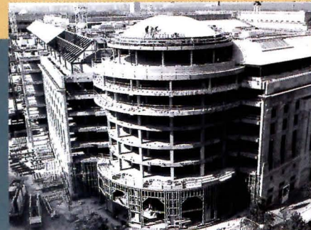
Pennsylvania Avenue rotunda being built.
