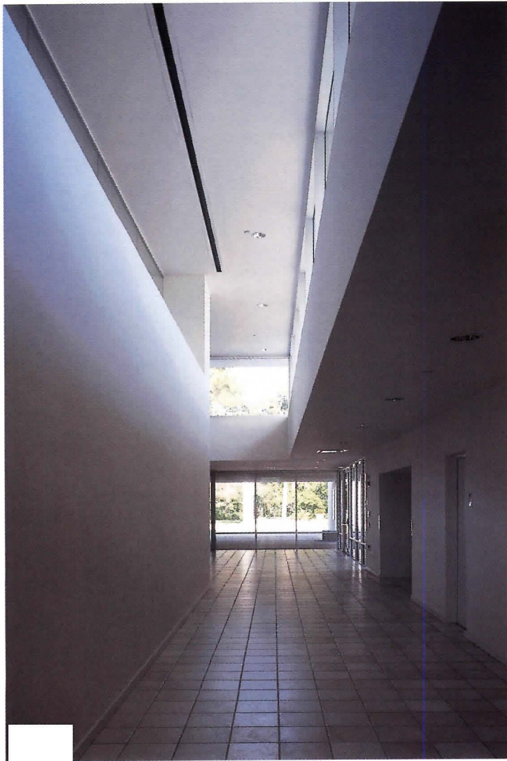
An interior corridor in the new parish hall (above), which leads from the main room to
