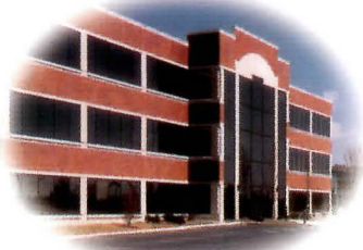
Professional Services Building, Allentown, PA
