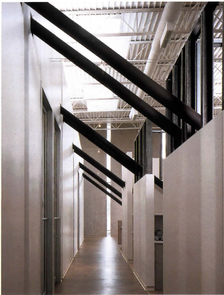
A blue-collar aesthetic prevails in the interiors, with roof decking, bar joists, and air ducts all exposed. Site constraints forced the angled bracing pipes indoors on the south wall (left and opposite), turning them into dramatic elements that define offices, conference rooms, and even the reception desk in the open office area.
