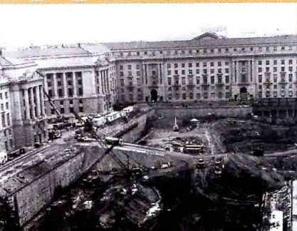
Preparing the site for construction.
