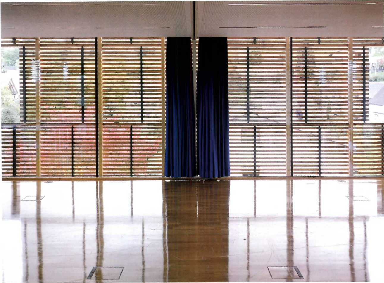
Horizontally movable wooden slats provide a flexible facade (above). The wooden lattice is about two feet away from the building's glass exterior (below), giving the building a multilayered face.
