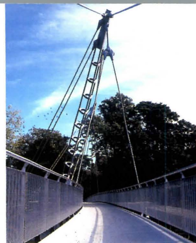
The slender cable-stay bridge at Maidstone (left) spans both a river and its floodplain. The cables are strung from two lacy masts (above).
