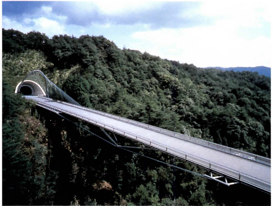
I. M. Pei's Miho Museum footbridge in Japan conducts visitors from a tunnel across a 400-foot span over a canyon approximately 100 feet deep.
