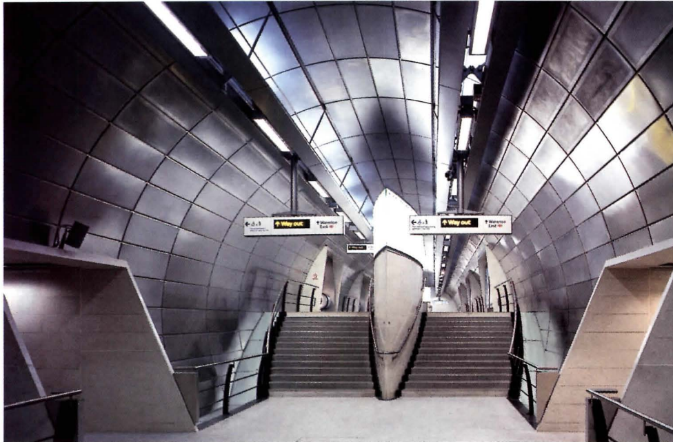
Left: At Southwark Station, pylon-mounted beacons and stainless-steel panels evoke the orderliness of a submarine.
