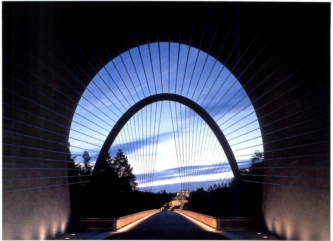
The 44 cables resemble a parting veil as pedestrians pass from the tunnel to the bridge (above). The posttensioned cables fan out (right) after passing through threaded rods in the arch (far right) and are anchored to the space frame.
