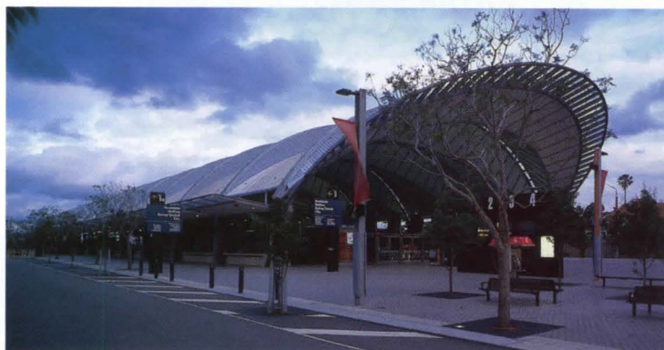
The Equestrian Centre by SJPH Design Partnership (top) and the award-winning Olympic Park Railway Station by Hassell Architects (bottom) are part of Sydney's rejuvenation effort.
