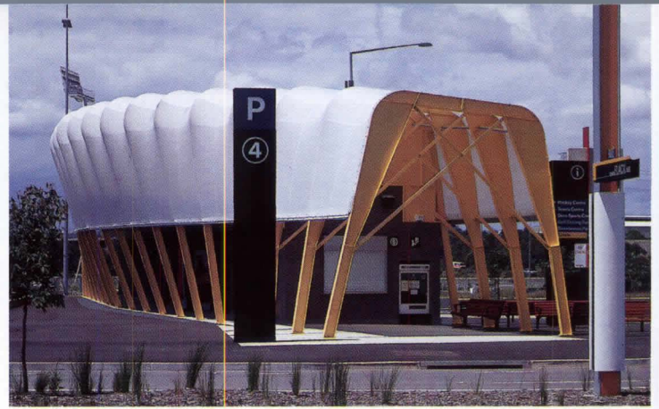
A gem among the Olympic buildings: one of Durbach Block Murcutt's three amenities blocks.
