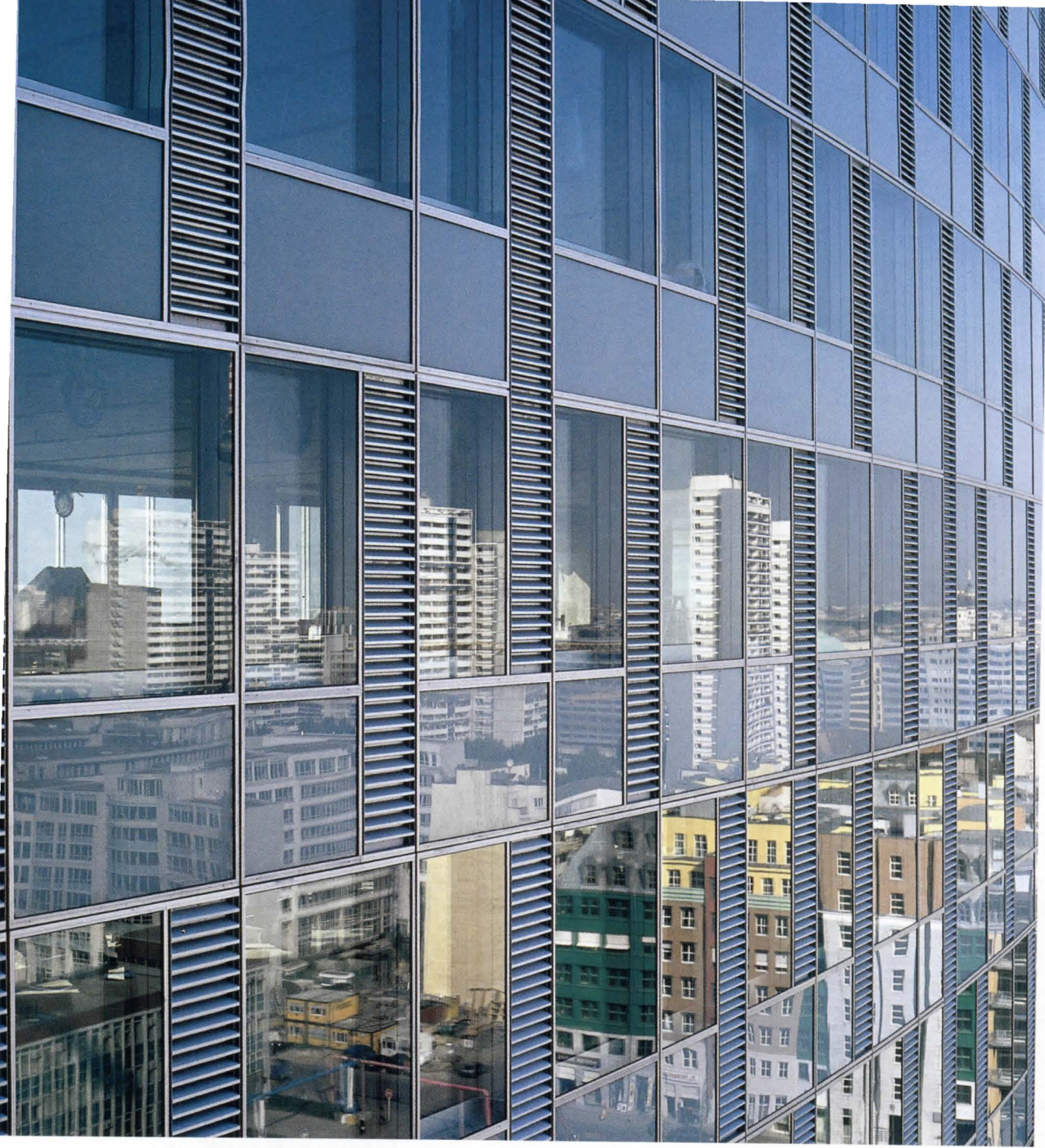
Louvers on the eastern, single-layer facade (left) admit breezes, usually to a corridor (bottom left). Alternatively, floors can be left entirely open (below, prior to move-in), giving users light and views from two sides.
