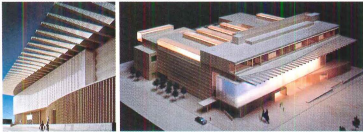
The Austin Museum of Art's curved wall of glass with aluminum fins (left).
