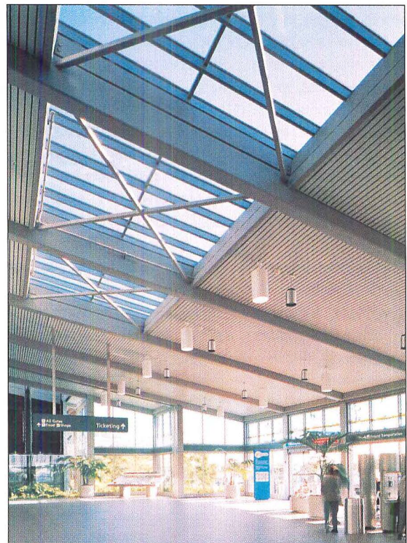
Photo: Sacramento International Airport, Terminal A Architect: Dreyfuss & Blackford Architects Photo: Cathy Kelly Architectural Photography A/D FIREFILM® II on structural steel.
