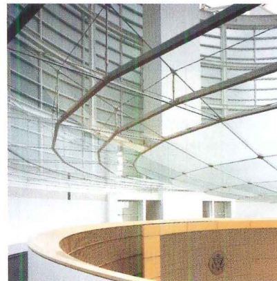
View from above the lens ceiling during construction (above). A visitor's view of the ceiling (below). Sprinkler pipe and cables were invisibly integrated (right).
