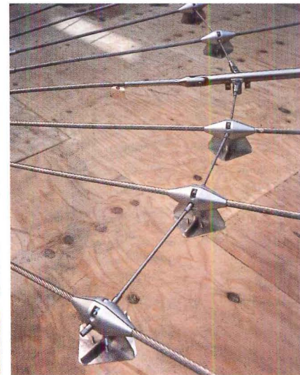
View from above the lens ceiling during construction (above). A visitor's view of the ceiling (below). Sprinkler pipe and cables were invisibly integrated (right).
