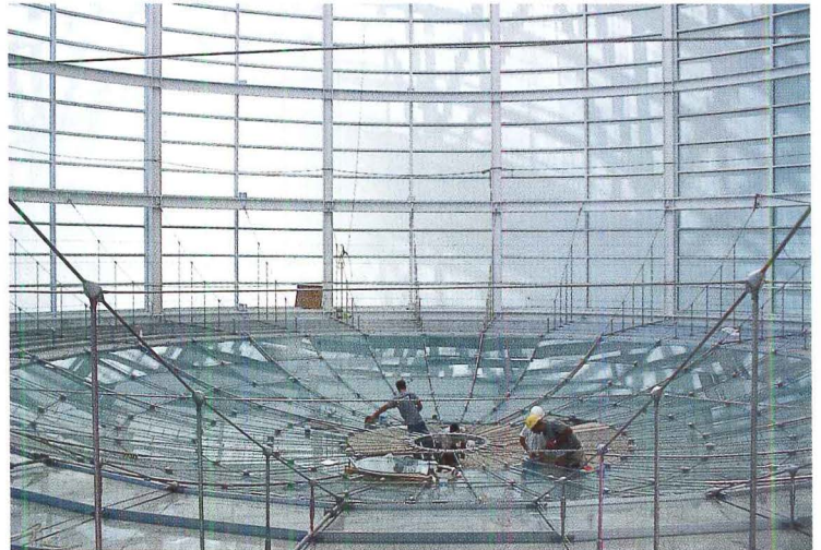
View from above the lens ceiling during construction (above). A visitor's view of the ceiling (below). Sprinkler pipe and cables were invisibly integrated (right).
