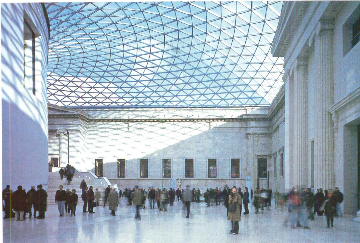
A glass-and-steel roof, weighing 1,000 tons, cover the 65,000-square-foot Great Court (left, below, and opposite). The Spanish limestone of the new building is Galicia Capri in a perfectly laid stack bond.
