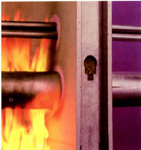
To achieve a desired fire rating for a partition or floor/ceiling assembly, all penetrations through that assembly must be treated with a firestopping material.
