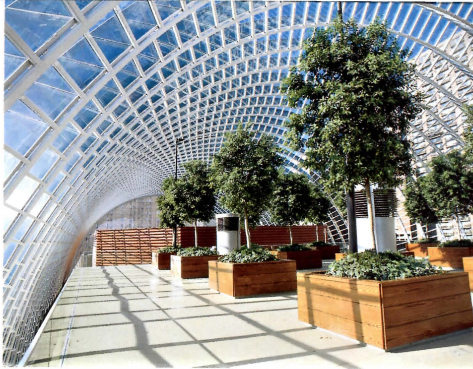
A roof garden with 16 planters sits atop the Perelman Theater, sheltered by the arched vault of folded-plate
