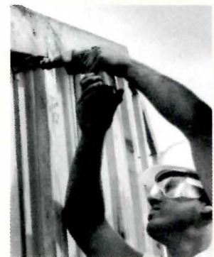
An aluminum breakaway clip is screw-attached to studs and framing. Under fire exposure, the clips break away, permitting the fire-damaged wall to fail while leaving the separation wall intact.
