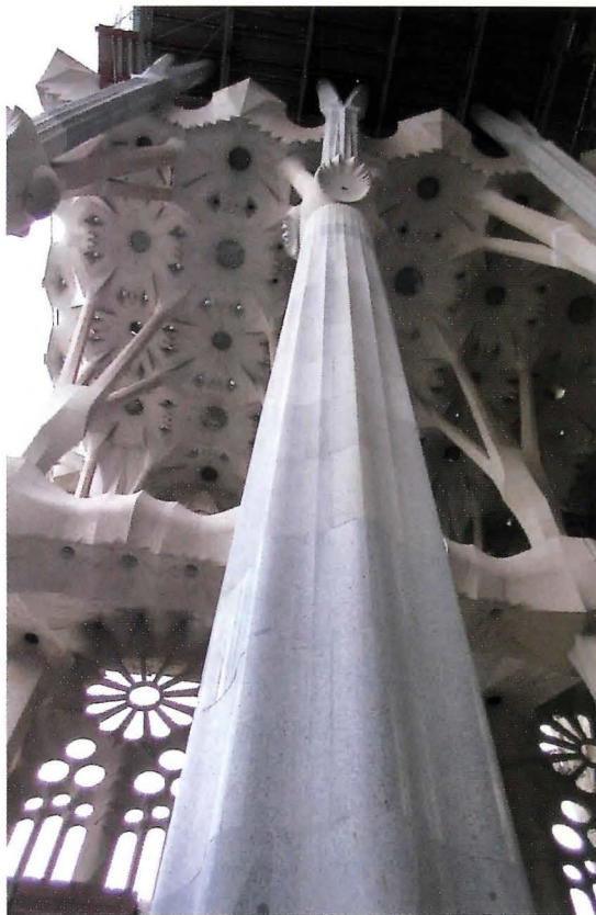
A column from Gaudí's Sagrada Familia Cathedral in Barcelona (above). Computer modeling illustrates the development of a single eight-sided column (top right), which shows a gradual addition of sine curves in cross section (bottom right). The sine curves undergo phase shifts as the column rises from base to capital.
