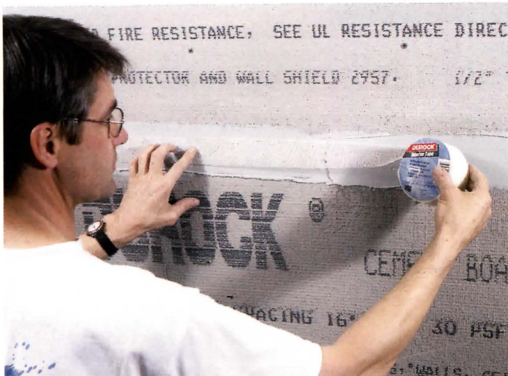
Cement board panels are made from approximately 20 percent recycled materials, including fly ash, a by-product of power plant emission control processes.
