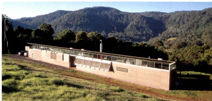
Work by Glenn Murcutt, all in Australia, includes (from top) the Marika-Alderton House (1994), in Northern Territory; the Magney House (1984), in Bingie Bingie; and the C. Fletcher and A. Page House (2000), in Kangaroo Valley.
