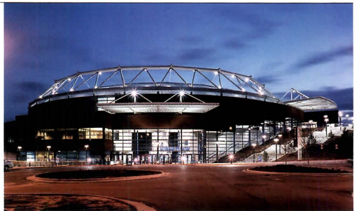
The Crown Coliseum in Fayetteville, N.C., is the first known tensegrity dome employing a conventional rigid structure of steel joists and metal deck.
