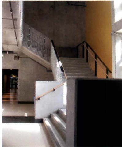
The reconstructed lobby stair.
