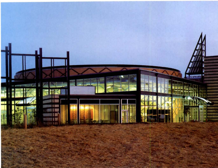
Prince Street Technologies Corporate Office Cartersville, Georgia, 1995
