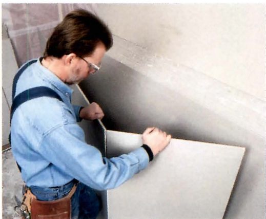
Gypsum board scores extremely high on nearly all sustainable design criteria. It is made from an abundant and non-endangered mineral (gypsum) and has low embodied energy. Drywall made from recaptured gypsum reduces landfill waste resulting from fossil-fuel power plant generators.
