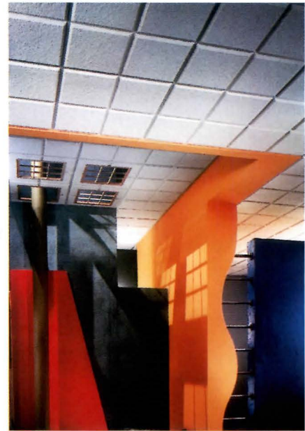
Most acoustical ceiling panels consist of approximately 40 percent mineral wool, which is usually made from slag, a by-product of steel manufacturing. The use of slag eliminates the need to mine and process naturally occurring materials, while reducing landfill waste.
