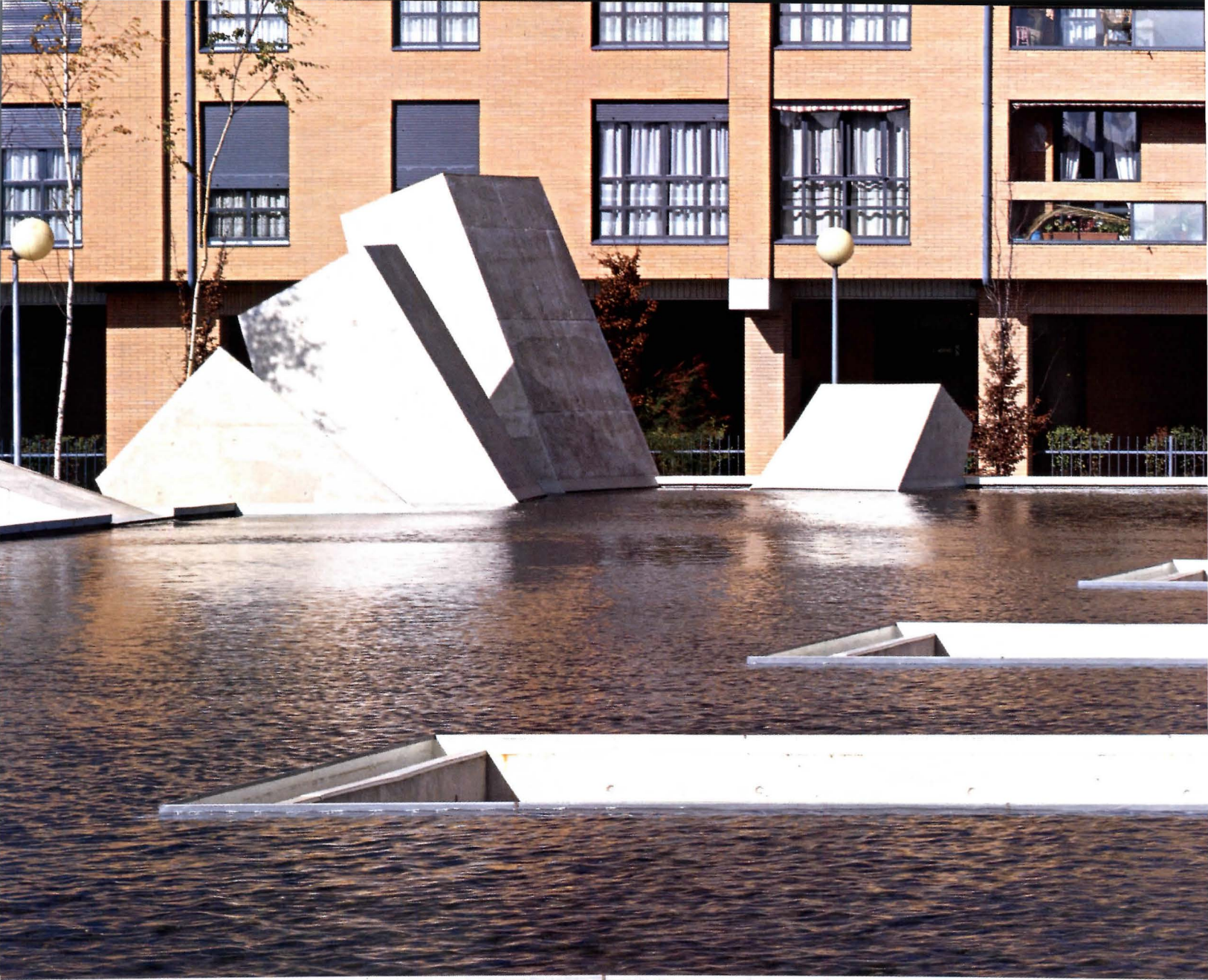
Sunken courts within the reflecting pool (above) bring daylight to vigil rooms below. Each court has its own small pool (not seen). Concrete “fingers” (above left) call attention to an entry ramp to the building and bring light into a chapel below. Apartment blocks overlook the project on one side, the river on another.
