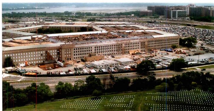
Over 500 mechanical equipment rooms are controlled by the Pentagon's EMS.
