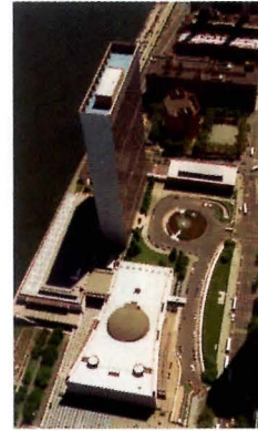
The United Nations will renovate its facilities.
