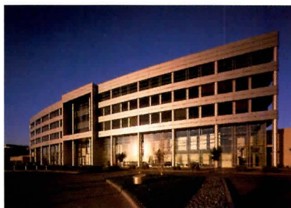
The LEED-certified Premier Automotive Group headquarters building in Irvine, Calif.
