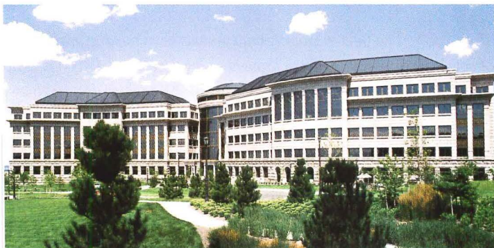
The all-precast structural systems for Starz Encore Headquarters, Englewood, CO includes double tees, inverted tee beams, shear walls and loadbearing precast walls. The system is a common approach to design in the Rocky Mountain region. Architect: Barber Architecture.
