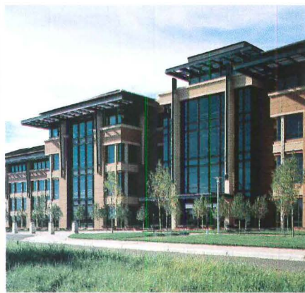
Two enormous portals that can be read from a distant highway mark the Merrill Lynch corporate office entrance in Englewood, CO. Architectural precast structural units with a finish mimicking Colorado red sandstone contrast with buff colored accents. Architect: Thompson, Ventulett, Stainback & Associates.
