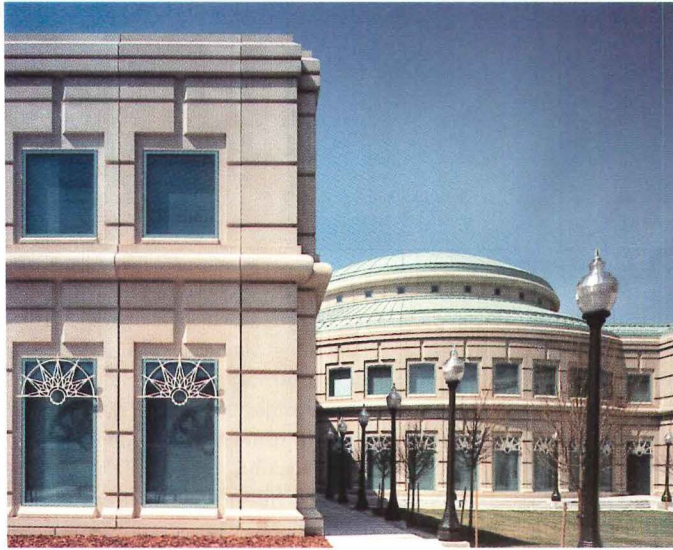
panels on loadbearing panels at Municipal Justice Center, Aurora, CO.
