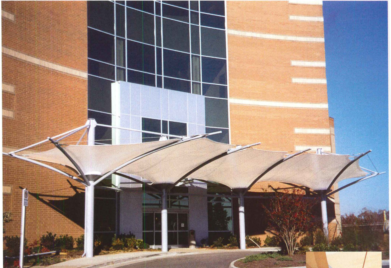
Tension structure in Knoxville, Tennessee, with painted steel frame and Ferrari brand fabric membrane
