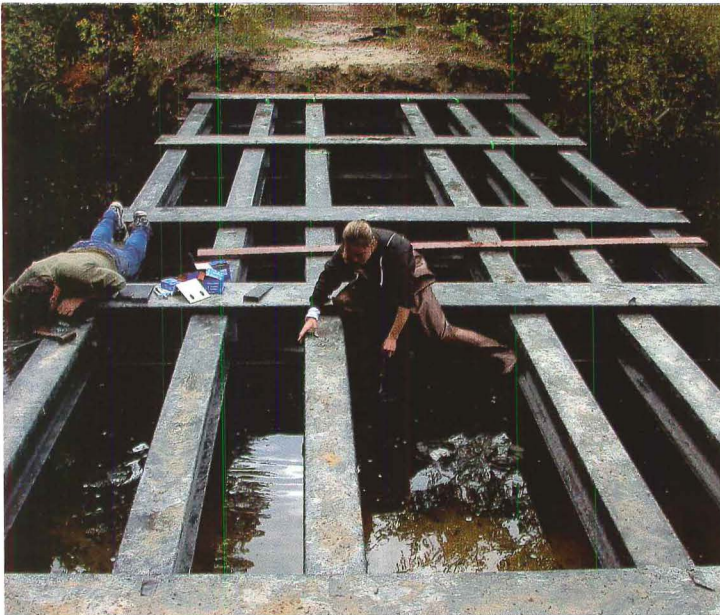
Researchers at Rutgers University building a bridge that will be strong enough to support a 25-ton truck out of plastic I beams and tongue-and-groove plastic decking developed at the Center for Advanced Materials.
