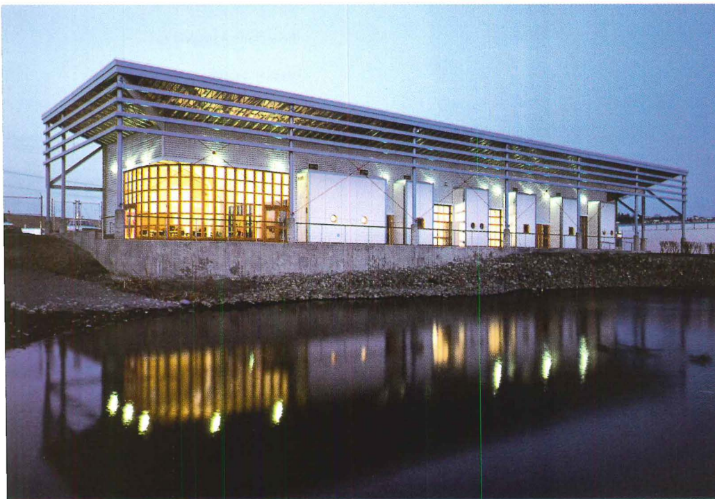
Marine Technical Facility, Seattle Central Community College Seattle, Wash., 1987
