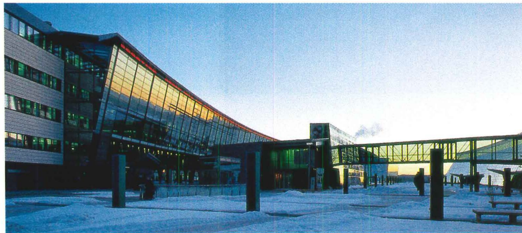
A long, narrow profile like that of the Telenor headquarters building is a common feature of sustainable design. If the building is oriented in the right direction, this form allows natural light to fall deep into the interior. Telenor says there is only about one lightbulb used per employee at Fornebu.
