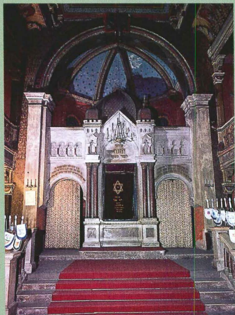
The principal facade (top) and the ark and its setting (above) as they appeared before restoration. The prayer hall ceiling was blackened by decades of neglect. The synagogue interior and exterior were still intact and thus required renewal of surfaces and finishes rather than significant reconstruction, apart from extensive repairs to the roof.
