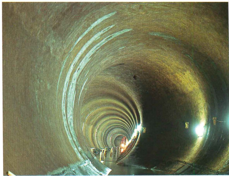
A spillway (top) that controls the level of Lake Gatun can also be seen in an aerial view (opposite). A ship in the lock at Miraflores (bottom left) and the culvert that supplies water to it (bottom right).
