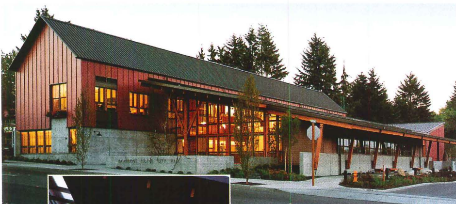
Bainbridge Island City Hall Bainbridge Island, Wash., 2000
