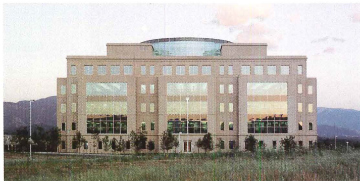
A bold sculptural form centering on a circular glass-topped atrium defines the Shepard's/McGraw-Hill World Headquarters in Colorado Springs, CO. The all-precast system offered the lowest cost and fastest construction schedule of several examined approaches. Architect: Barber Architecture.
