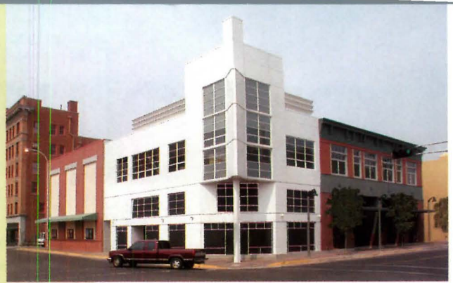
This retail and office building, by Moule & Polyzoïdes, gives prominence to an important corner and wraps a cinema's blank walls.
