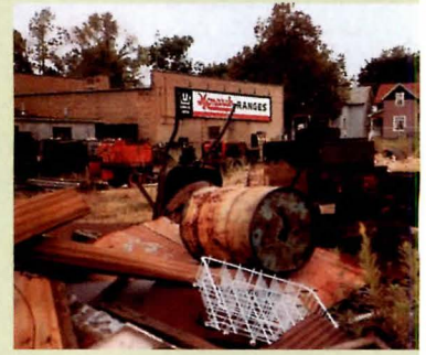
Architect-developer Martin Sell facilitated the cleanup of the Monarch Range industrial site (above). He divided the property into parcels (plan) for development.
