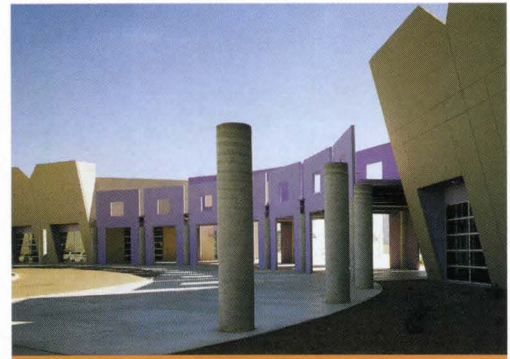
1990s It goes in pieces: Tilt-up construction allows low-rise concrete structures to be built without formwork, often in less than a month.
