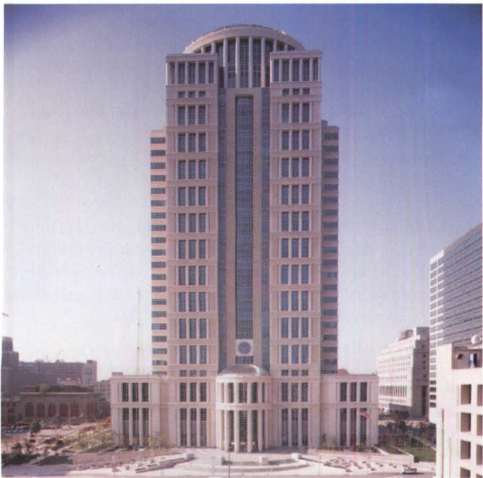
The Egleton Center, a Federal building in St. Louis, Missouri, is a 27-story structure of precast panels colored with CHROMIX Admixtures in a custom color that also matches the surrounding hardscape.
