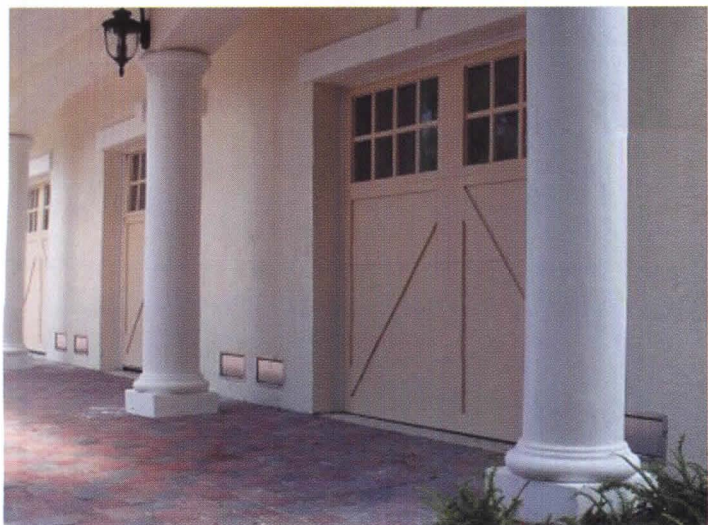
Flood VENT™ Installation
