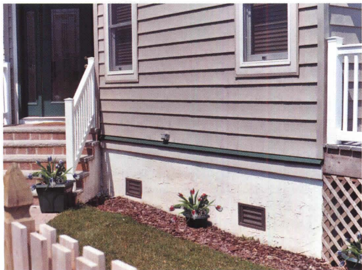
Smart VENT® Installation
