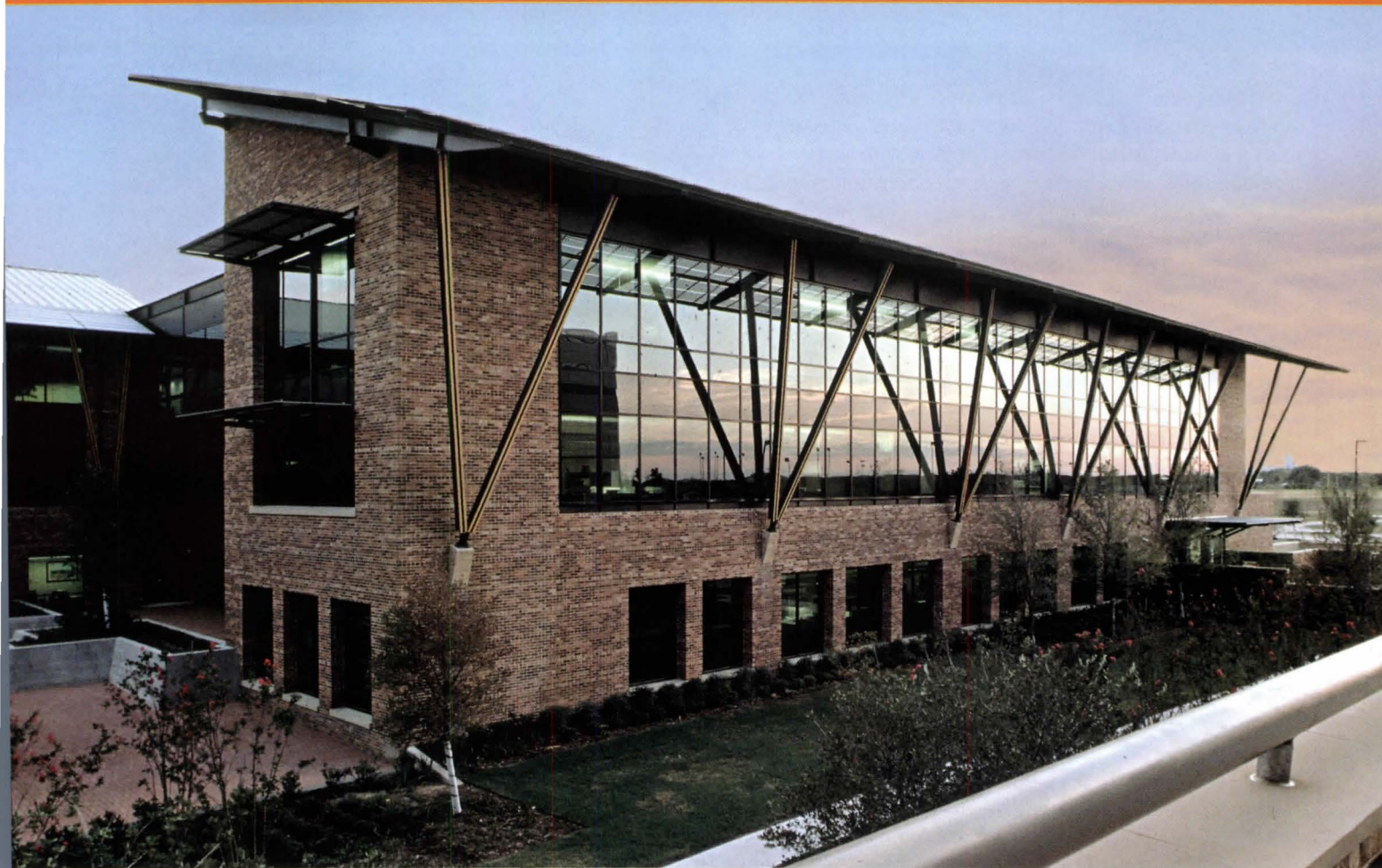
Arlington Northern Santa Fe Road Headquarters Worth, 1996
