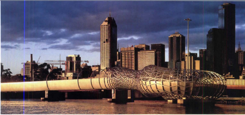
The Webb Bridge was towed on a barge to the site on the River Yarra.
