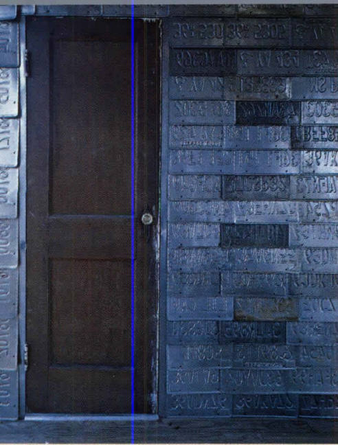
Detail of one of the Pods (note wall made of license plates), Newbern, Ala., Rural Studio. 1997–2001.
