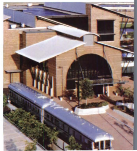
Burlington Northern Santa Fe Railroad Headquarters (with KVG Gideon Toal) Fort Worth, 1996
