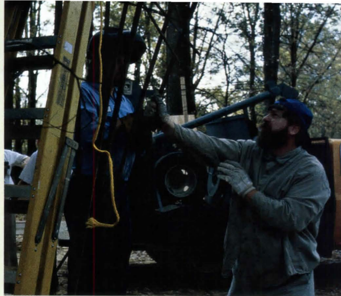
Sambo working on the tractor shed, Flautt House, Greenwood, Miss., Mockbee Coker Howorth Architects, 1988.
