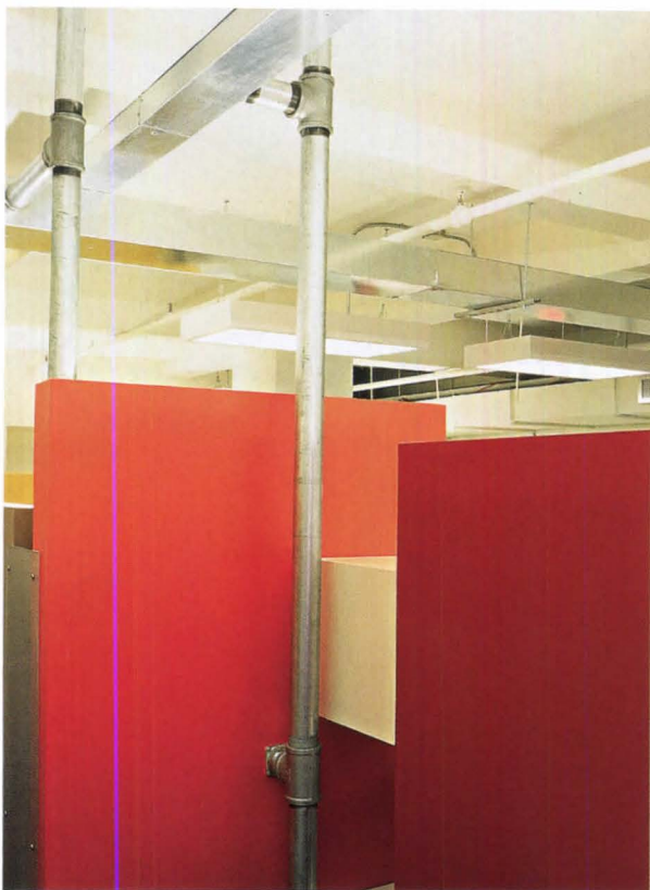
Galvanized-steel pipes convey power cables to workstations (above left and right). Left unfinished and exposed, they join laminated-wood shel-
