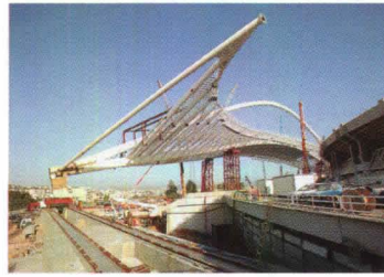
Olympic roof slides into place.
