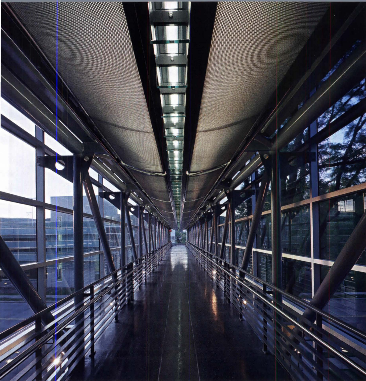
The ceiling (above), on which slightly bowed, perforated-steel screens and a spine of crystal louvers are mounted, adds to the luminous effect of the elevated bridge. The long stair (right), with well-proportioned pipe rails and flat balustrade rails, creates a grand entrance at the south end, where the bridge connects to Corning's office buildings.
