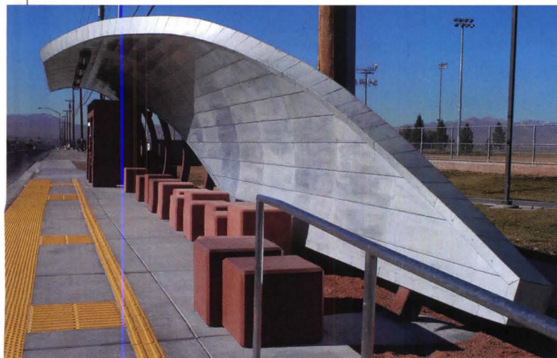
Assemblage Studio Architects of Las Vegas designed a whimsical shelter for a state-of-the-art bus system to be introduced this summer.
