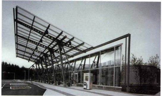
The glass canopy of the visitors' pavilion (above) shelters a triangular glass structure attached to a round concrete bathroom core. The skyway bridge (opposite) cantilevers at the north end (below), next to the parking garage.
