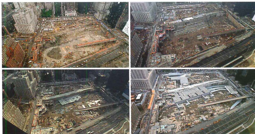
Project Rebirth uses time-lapse photography to capture the rebuilding of the World Trade Center. The site went from a hole (top left) to a construction zone (bottom right).
