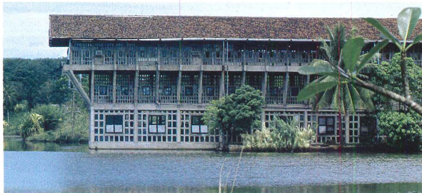
Natural ventilation cooled all of Bawa's buildings, including the Steel Corporation headquarters in Orawela (left), the Ena de Silva House in Colombo (below left), and the State Mortgage Bank in Colombo (below right).
