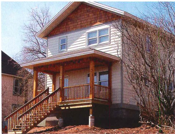
MasterFit Frames (right) are shipped to a site and assembled with joinery included in the kit. The house above was built by seven women enrolled in a carpentry-training program in Duluth, Minnesota, who had only one week of experience.
