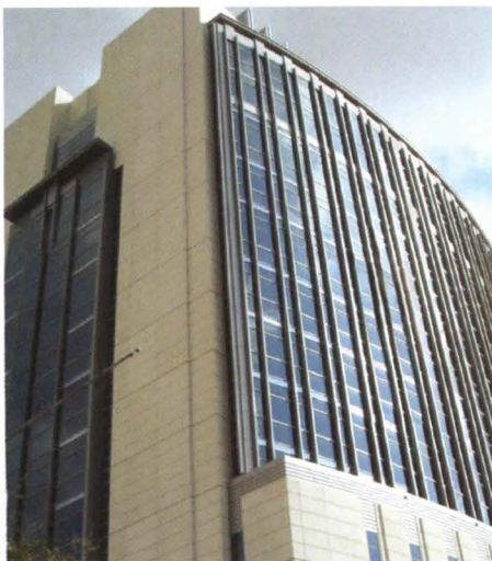
United States Federal Courthouse, Jacksonville, Florida. Architect: HLM Design. Photo courtesy of Solutia Inc.
