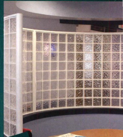
Round caps finished off the ends of this radius wall perfectly. Aluminum mulls were used to connect the three radius walls together, while a flat cap mounted the units to the top of the curved wall.
