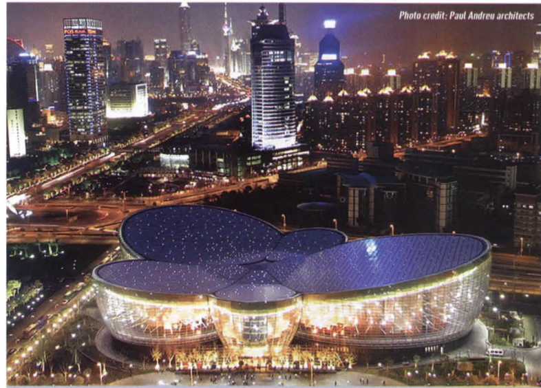
Shanghai Oriental Arts Center, Shanghai, China Metal mesh screens were laminated between structural interlayers to provide glare reduction and daylighting benefit. Architect: Aeroports de Paris, Paris
