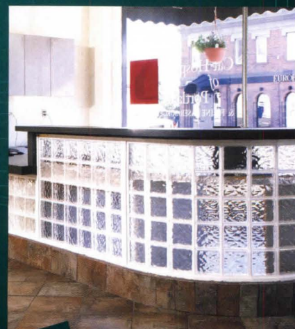
Aluminum mulls were used to connect these flat panels and radius walls together. A flat cap and mounting channel were used to mount the units to the base and the walls. Flat caps were also used to connect the desktop to the top of the panels.
