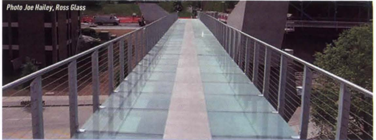
Holmberg Pedestrian Bridge, Chattanooga, Tennessee The use of laminated glass with advanced polymer interlayers allowed strength and transparency in this key waterfront redevelopment project. Architect: Derthick Henley & Wilkerson Architects, Chattanooga
