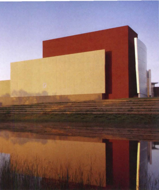
Legat Architects' Lake Zurich High School Performing Arts Center in Lake Zurich, Illinois (left), represents a resurgence in school performing arts architecture. Leaflike metal walls and abstract concrete plates emphasize the building's artistic function (top and bottom). Acoustical wood panels and sculptural wood reflector panels articulate the dynamic interior (middle).
