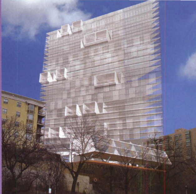
LakeBluff Tower, Milwaukee, Wis., 2005 This mixed-use office and town-house building is oriented to have an open-view corridor framing Lake Michigan and Veterans Park. Four town-house units on the ground level have unobstructed views of the lake and city skyline.
