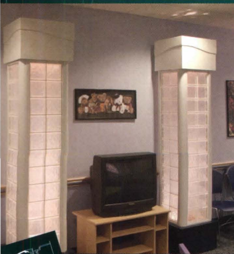
90-degree corner caps were used to connect four acrylic block panels together to form decorative, lit towers. The panels were mounted to the base and top piece with flat caps.
