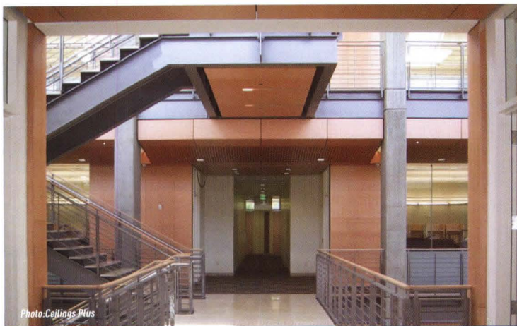
Photo: Ceilings Plus Book-matched, quarter-cut eastern hard maple was selected by Yost Grube Hall Architecture for the Kelly Engineering Center at Oregon State University in Corvallis, OR. The project is expected to receive LEED Silver certification.
