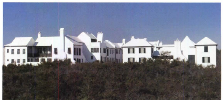
The houses of Audubon Village (top) are reinforced against wind; concrete stilts allow them to stand above potential flooding. Recently completed buildings in Alys Beach (above) mask their defenses in the style of new urbanism.
