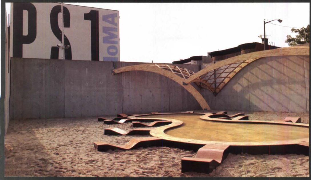
OBRA Architects' courtyard canopies, constructed of plywood and polypropylene, shelter hundreds of visitors to P.S.1's Saturday parties, when the crowds are avoiding the sun (above) or wading through one of the wood pools (below).
