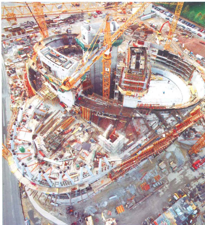
The museum consists of stacked trefoil-shaped elements, each with two propeller-shaped spaces—one for vehicles and the other for historical displays.
