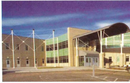
Precast concrete panels can provide a traditional brick appearance or a more contemporary look, as seen here at Columbine High School in Columbine, Colo.
