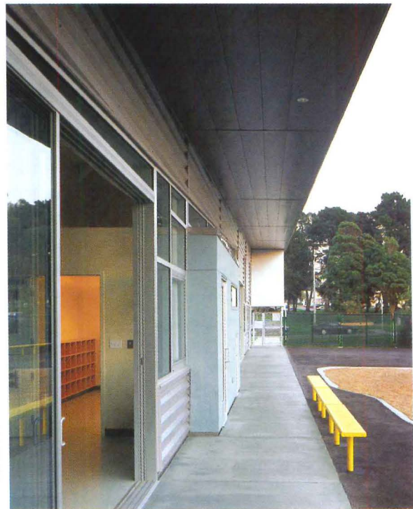
Sliding glass doors in the south facade (above and right) open to a landscaped play area, where aromatic plants and varying surfaces encourage sensory exploration. Window headers echo the slope of the roof. Corrugated metal panels and large glazed openings contrast with stucco surfaces and punched openings.
