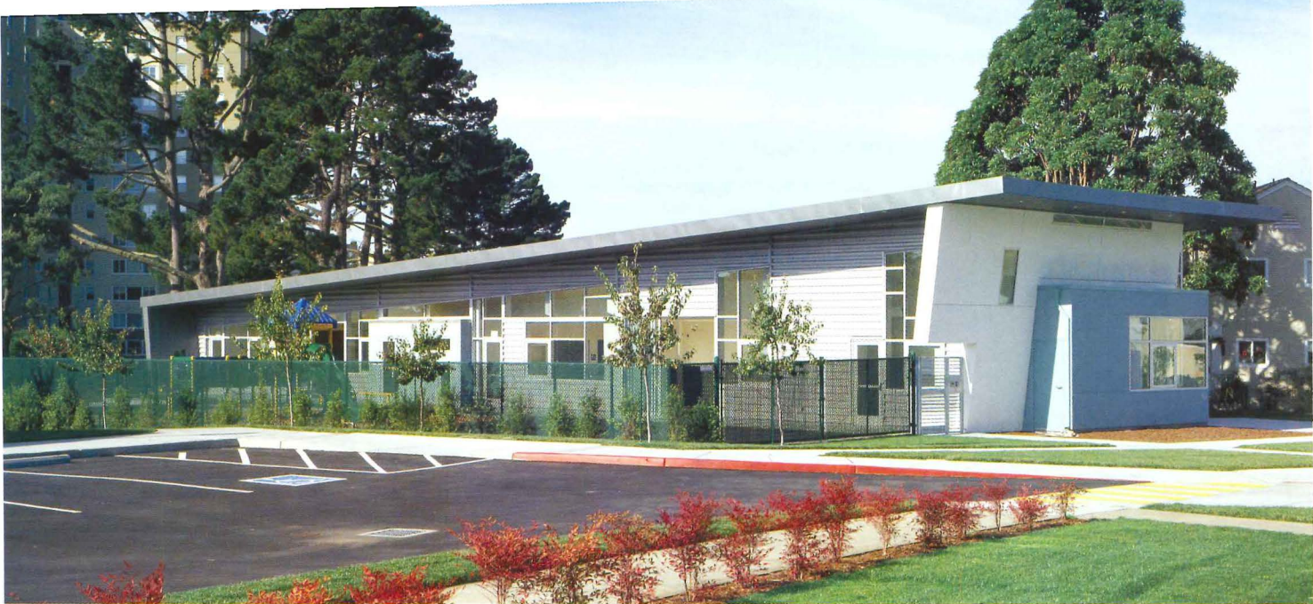
Sliding glass doors in the south facade (above and right) open to a landscaped play area, where aromatic plants and varying surfaces encourage sensory exploration. Window headers echo the slope of the roof. Corrugated metal panels and large glazed openings contrast with stucco surfaces and punched openings.
