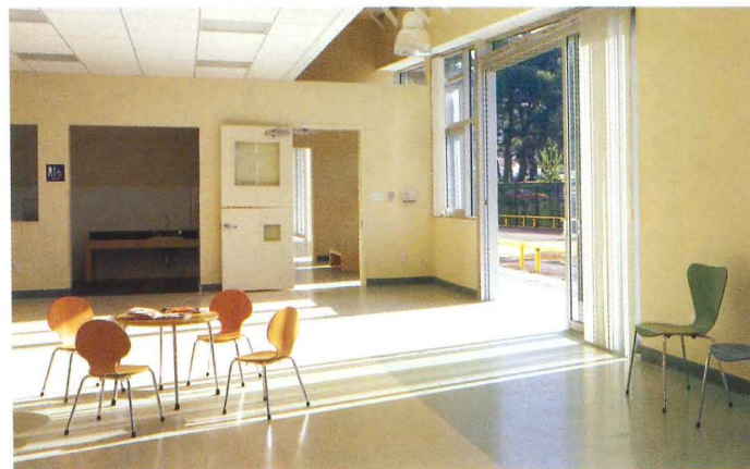
A stained concrete playground patio (above) transitions to vinyl classroom floors inside the building (left). Differing colors of the vinyl flooring material and a ceiling soffit distinguish classroom space from a circulation zone.
