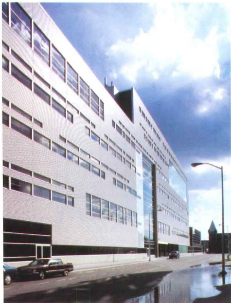
The architect used dynamically arranged fenestration and a variety of materials for the building skin, including brick, glass, and metal panels.
