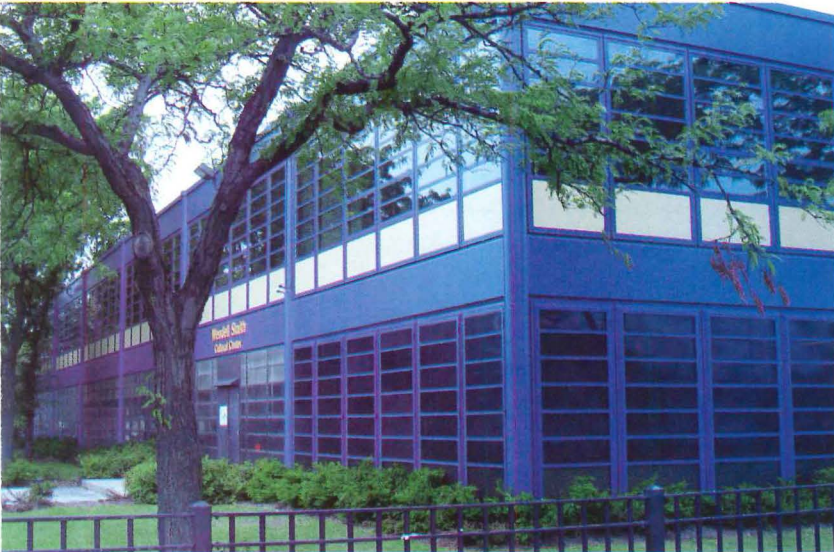
Graham school windows help control the sun with low-e glazing, internal blinds, and multiple operating systems for good ventilation. (Shown: Lincoln High School, Denver.)
