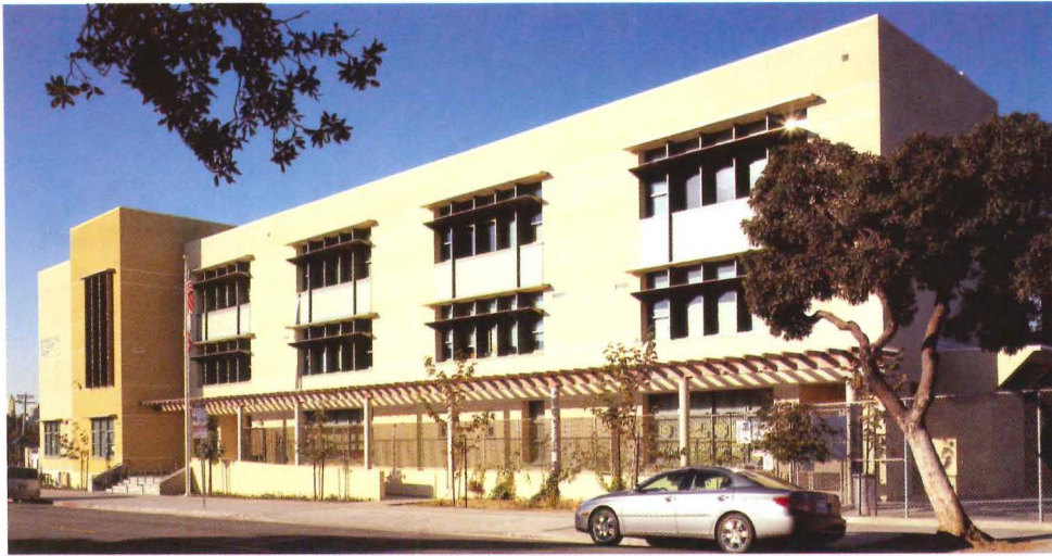
Harley Ellis Deveraux, an architecture and engineering firm, and Greenworks Studio, a sustainable design consultant, recently completed Charles H. McKim Elementary, a CHPS school in Los Angeles.
