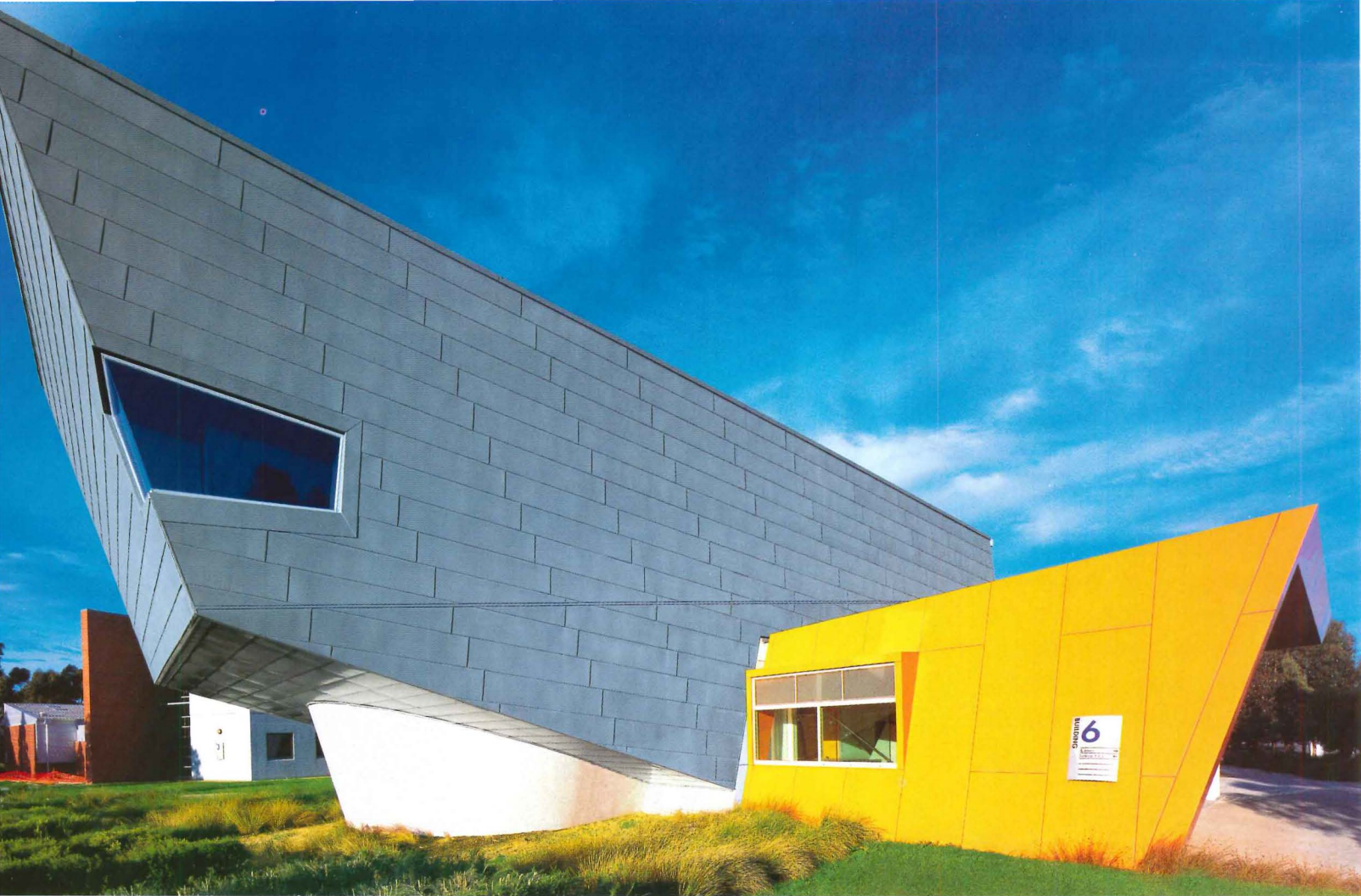
New Lecture Theatre, Victoria University, Werribee Campus, Werribee, Victoria, Australia; Architect: Michael McKenna Pty Ltd, Melbourne, Australia
