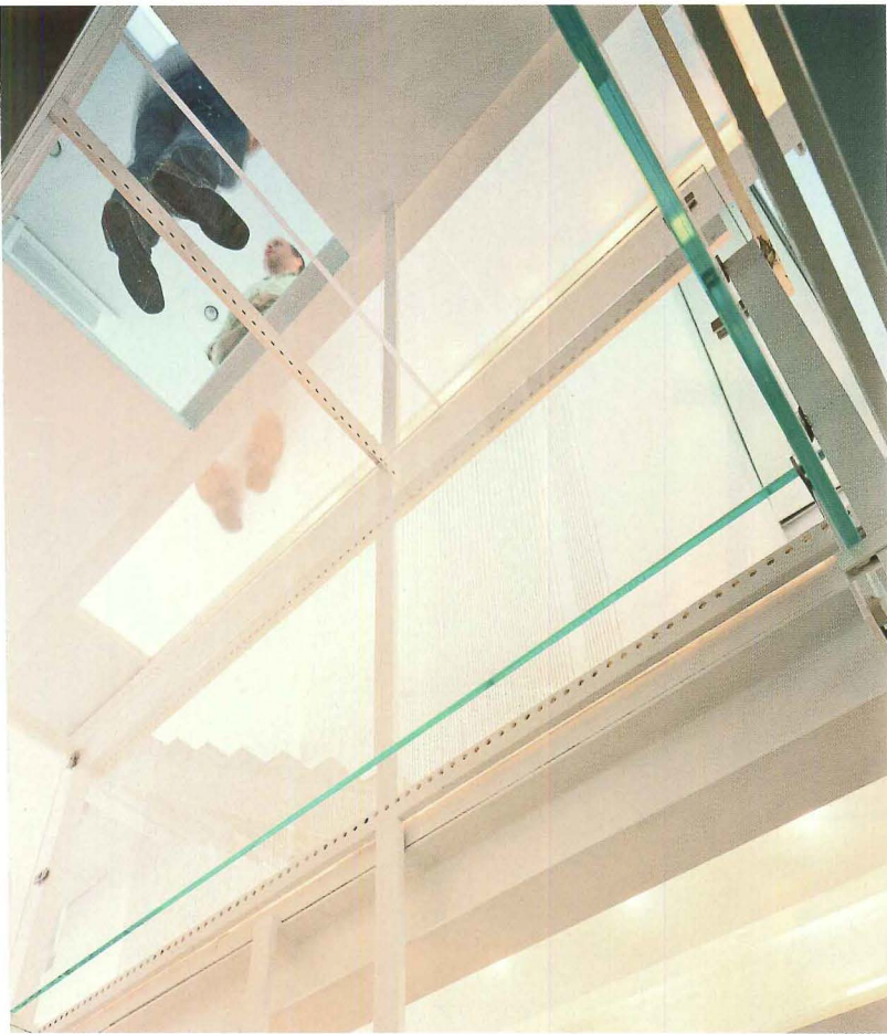
After removing a dumbwaiter, the architects sealed off the shaft with clear acrylic (left). They installed a new opaque-solid-surface master tub (below) in place of the original transparent one west of the master bedroom.
