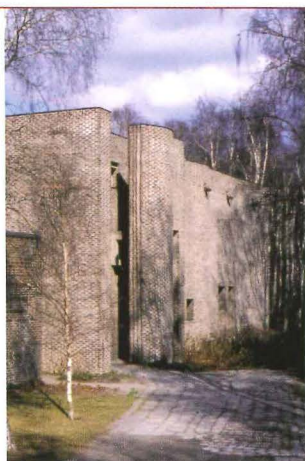
Sigurd Lewerentz dictated the placement of each individual brick during construction of his 1956 St. Mark's Church (above and left), outside of Stockholm.
