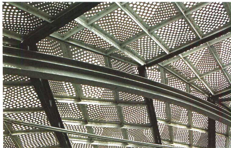
548 W. 29th St., New York City, 2009 Near the High Line in Chelsea, this 12-story condominium building will cantilever 12 feet over its neighbors on both sides. It has a folded metal facade with panels of varying height.
