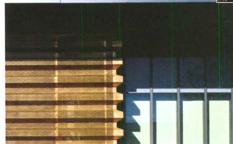
A copper scrim at the Illinois State Emergency Operations Center screens the interior but allows daylight into the building and provides views of its wooded site.
