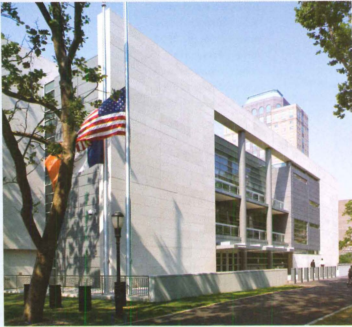
Designers of New York City's OEM worked with the structure of an existing building, moving its core from the center to the south elevation (above left). They used the new core as a screen (bottom left) by carving out terraces and the lobby (middle left). The configuration allowed for a large, clear-span space for the emergency operations center (right) with its immediately adjacent situation room (above right).
