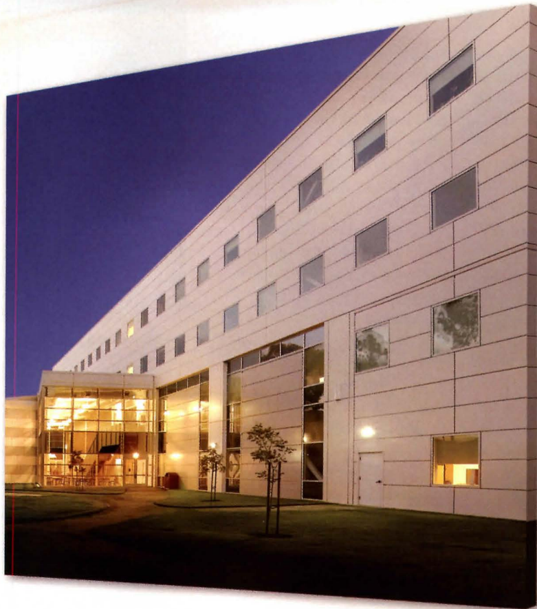
Business & Technology Center California State University VBN Architecture Formawall Dimension Series Insulated Metal Wall Panels FormaBond Metal Composite Wall Panels
