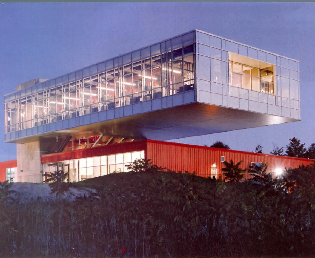
Lamar Construction Company, Hudsonville, Michigan For this small corporate headquarters outside of Grand Rapids, Integrated Architecture developed a 100-foot-long cantilever to lend the project presence from a nearby highway. The client also wanted to highlight its technical expertise through an ambitiously designed and constructed building.
