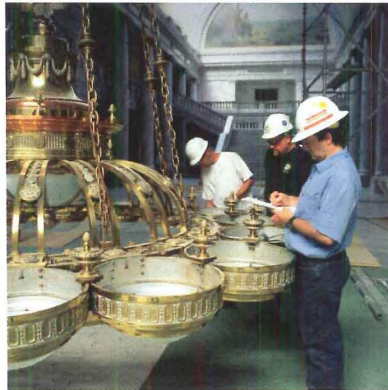
CUSTOM LIGHTING Utah State Capitol Salt Lake City, UT
