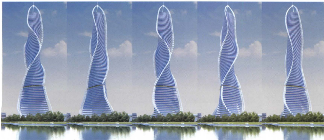
Because floors would rotate independently of each other, the building's shape would constantly change (above).
