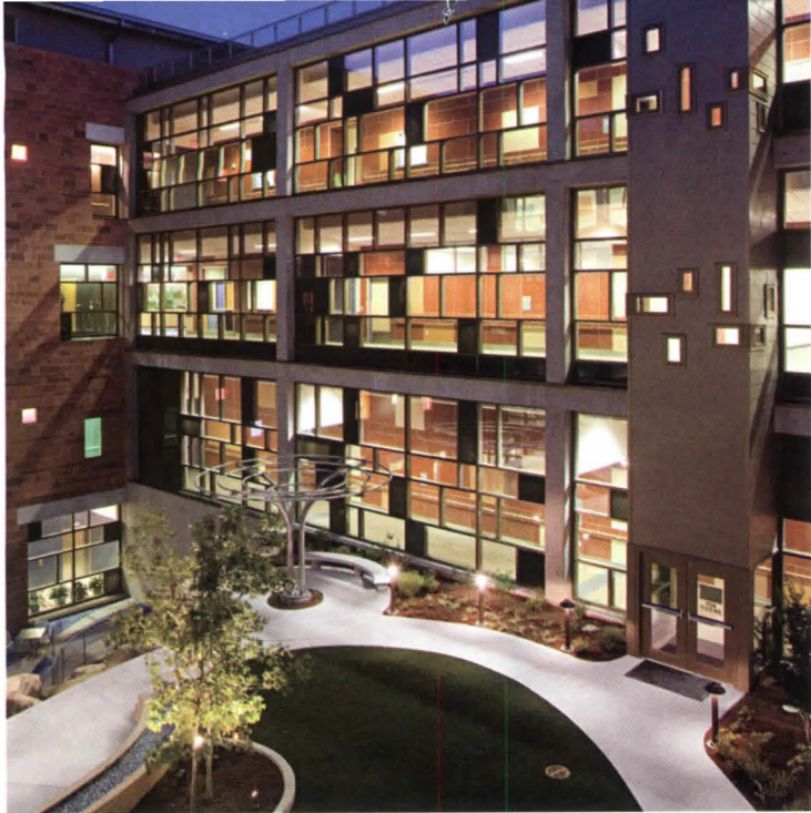
Dell's entrance tower acts as a landmark (opposite). The courtyards, most of which are accessible, serve as air intakes for the building (left and below).
