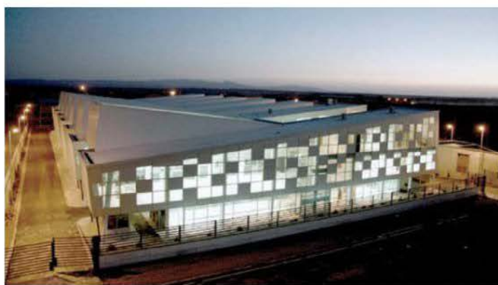
The panel factory scheme is based on a repetitive and alternating geometry.
