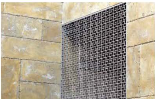
Clockwise from top left: Custom concrete sink and tiles; a central stair features custom hand-cast concrete wall panels and floor tile; a custom aluminum grille is set in a field of the stairwell's wall panels.
