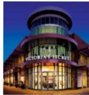
Victoria's Secret, Chino Hills, CA Architect: McCall Design Group Custom-engineered Storefront by Oldcastle Glass® Vistawall®
