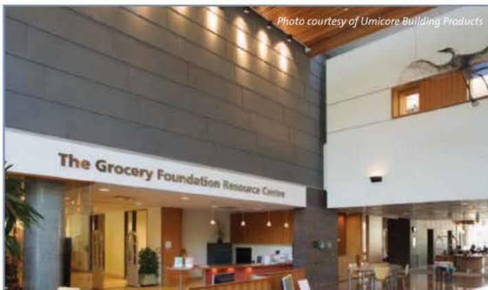
Bloorview Kids Rehab hospital in Toronto, Canada includes interior walls of zinc flatlock shingles. The hospital also has a zinc roof. Architect: Montgomery Sisam. Installer: Flynn Canada
