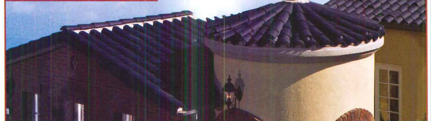
Solar tiles integrate with clay tiles for a seamless look.
