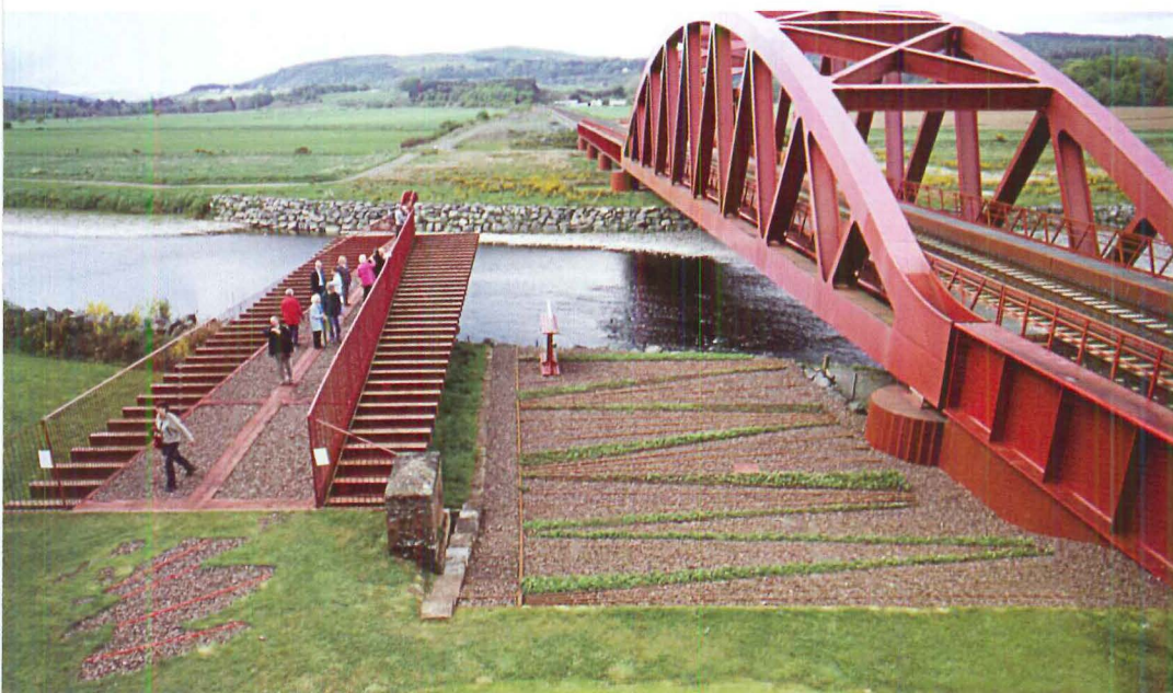
The bridge cantilevered from ruins of the old one (far left) now acts as a viewing platform. Between it and the new bridge is a real rail garden of rusted rails, red ballast, and strawberry plants.
