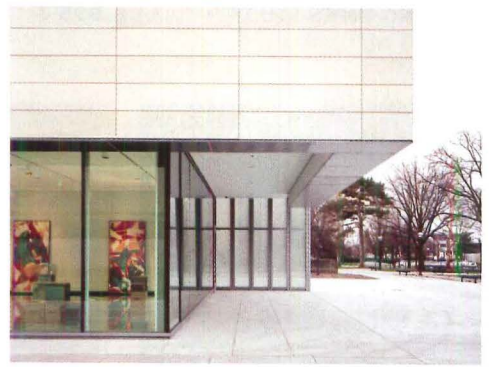
ABOVE: Much of the Frankel Wing's exterior is clad in Wisconsin-quarried "Tiger Stripe" limestone.
