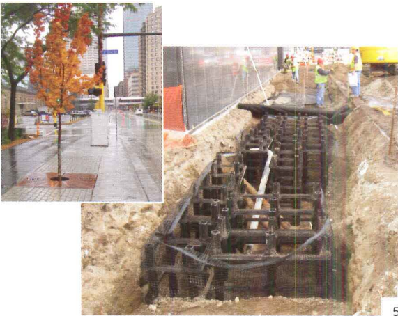
5 | PRODUCT Silva Cell Subsurface Tree Protection and Stormwater System MANUFACTURER Deep Root Partners deepproot.com
