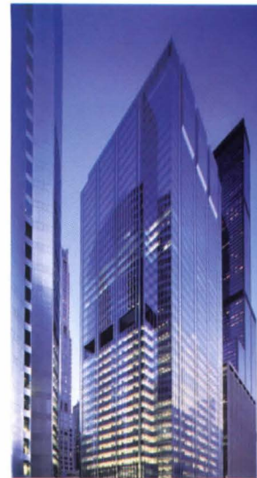
Custom Curtain Wall at 111 South Wacker designed by Goettsch Partners, custom-engineered by Oldcastle Glass®
