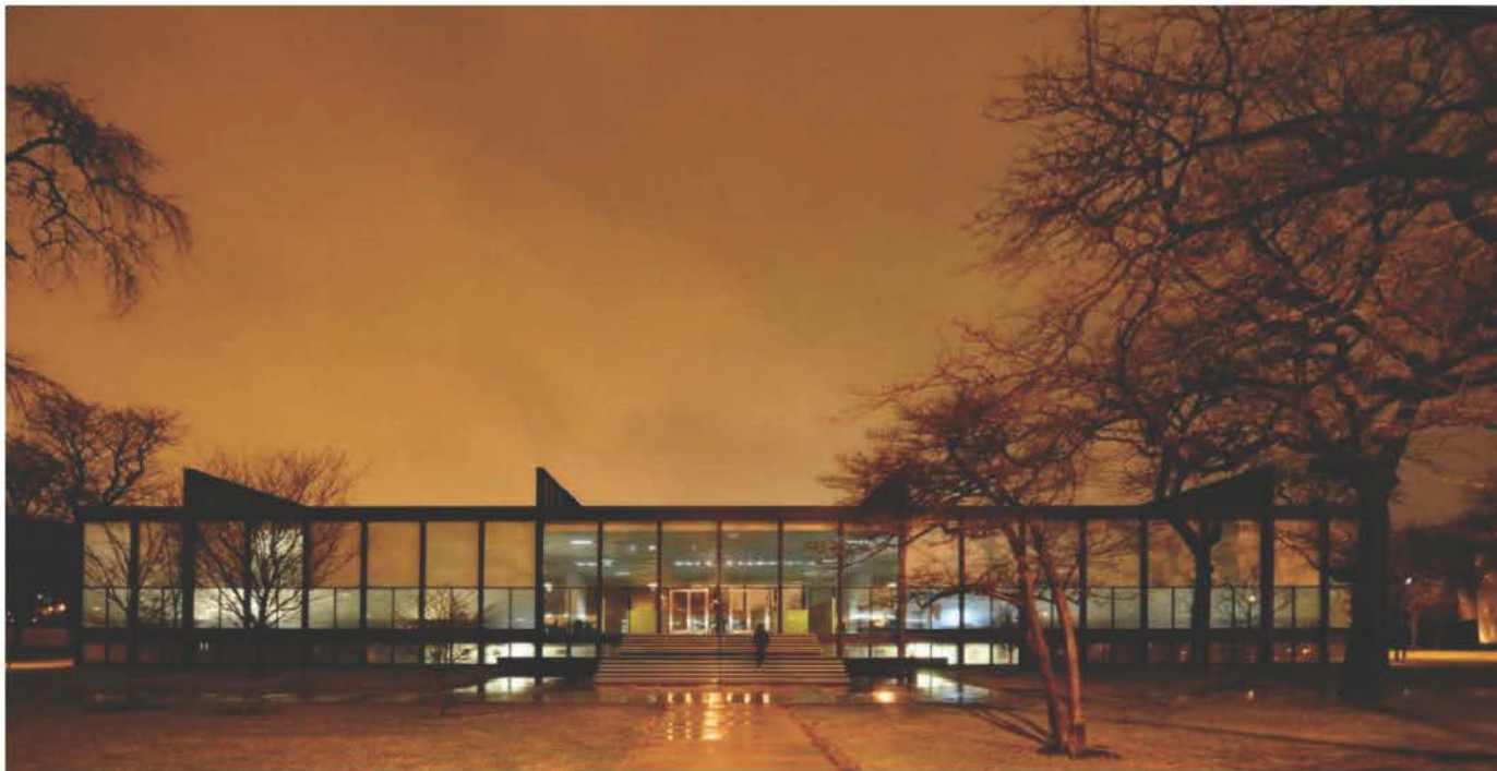
Illinois Institute of Technology's Crown Hall at 3 a.m. | Ludwig Mies van der Rohe | Chicago, Illinois | Submitted by splenert.
