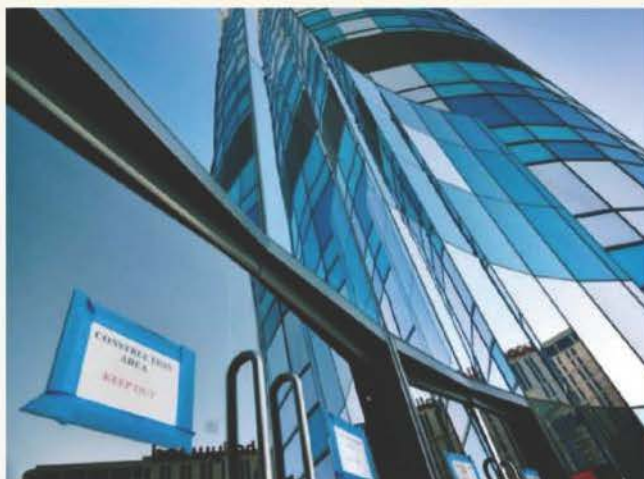
MGM decided to cap CityCenter's Harmon Hotel at 28 stories instead of the originally planned 49 after inspectors discovered a construction defect. Interior fit-out of the building has been delayed indefinitely.
