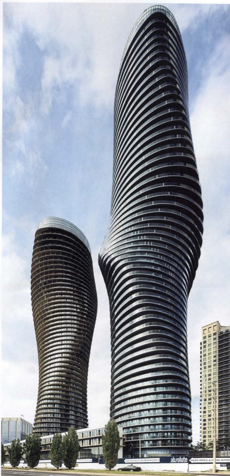
The 56-story “Marilyn” tower (foreground) and its slightly shorter sibling, both designed by Beijing-based MAD, contrast sharply with their more ordinary neighbors.
