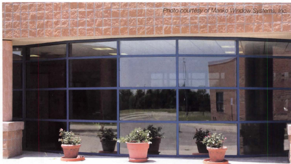
Single-story storefront system used in a common light commercial retail setting
