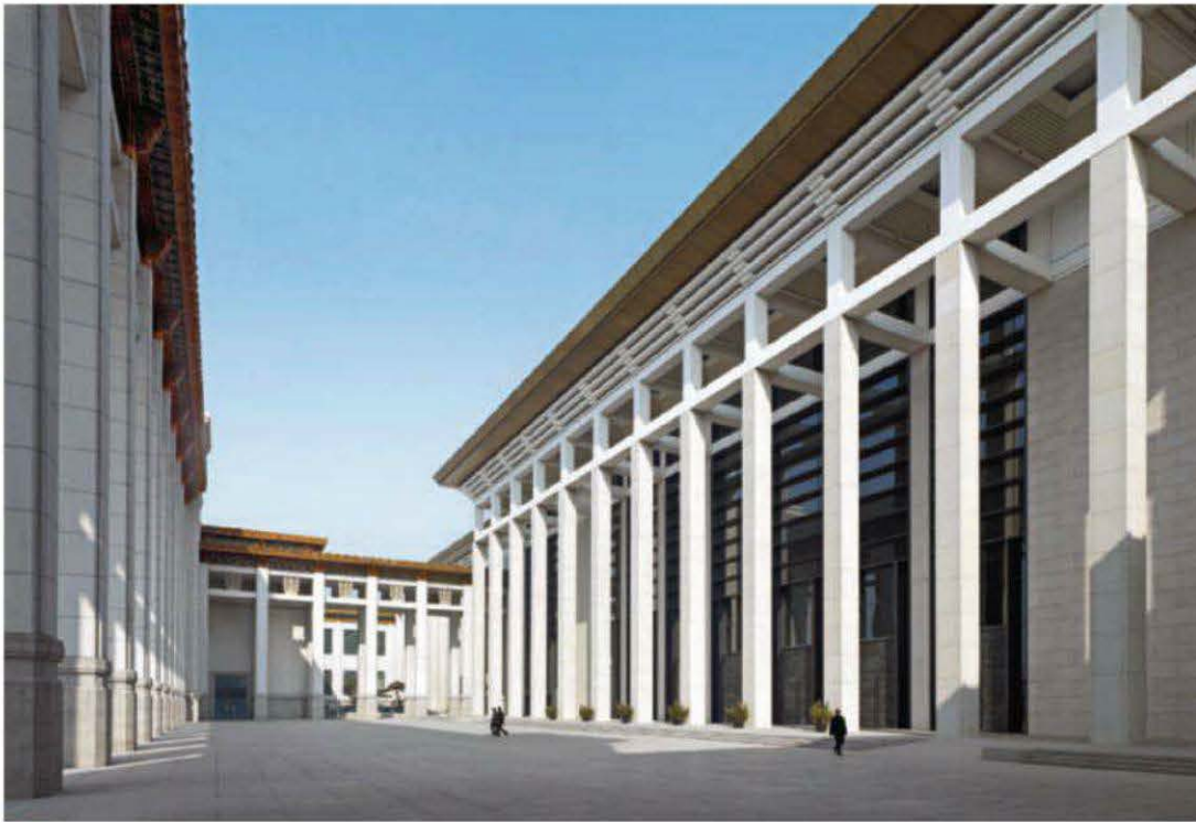
LEFT: The museum's historic and new (at right) facades are separated by a long, outdoor courtyard. OPPOSITE: Coffered ceilings, banks of stairs and escalators, and granite and cherrywood cladding add warmth to the otherwise empty Grand Forum.
