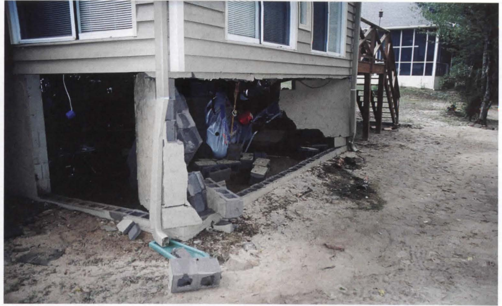
Hydrostatic pressures are extremely strong under flood conditions, and can shift, separate and even destroy foundations if not properly floodproofed.
