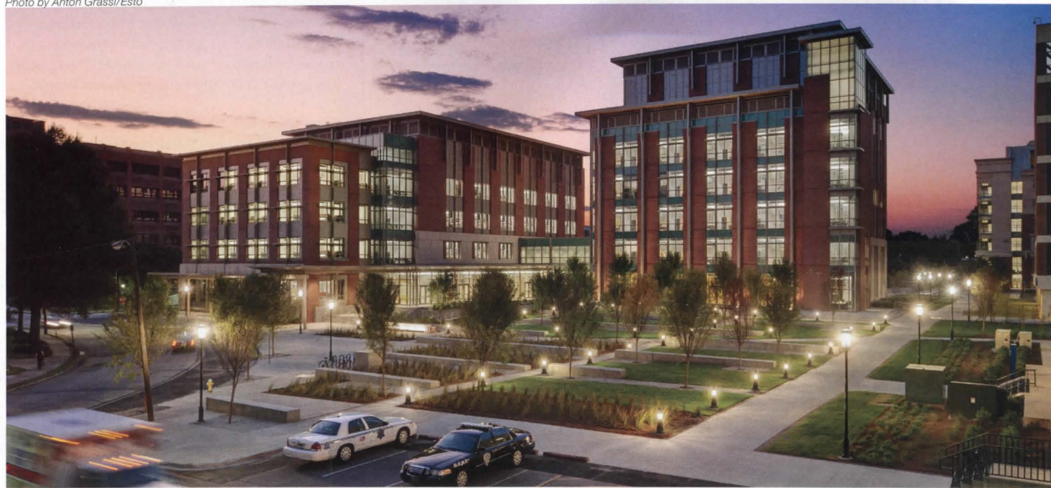
At the new James E. Clyburn Research Center, Charleston, South Carolina, foundation flood vents meet functional as well as aesthetic requirements.
