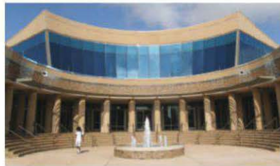
Controlling water penetration on campus buildings was important when designing a building that is clad in brick, glass, and precast concrete.
