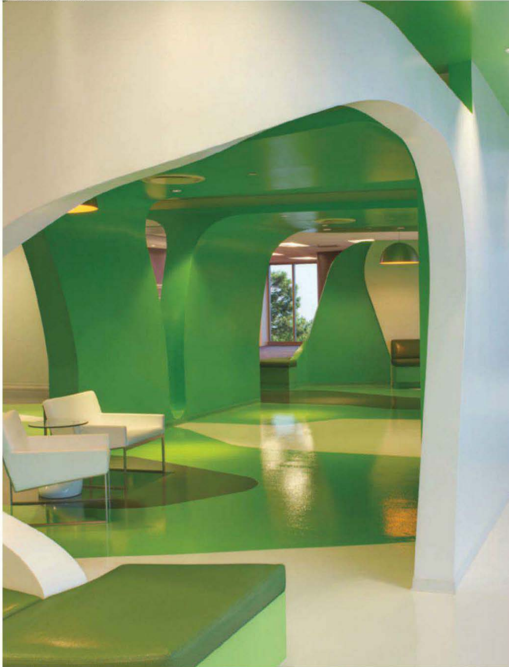
Decorative troweled epoxy floor unifies the design of a corporate office.
