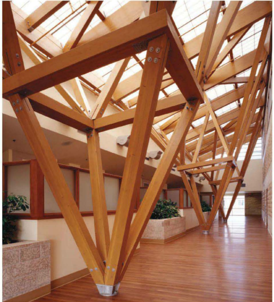
Thunder Bay Regional Health Sciences Center in Ontario, designed by Salter Farrow Pilon Architects Inc., was the first hospital in Canada to gain approval for the use of wood as a primary structural element.
