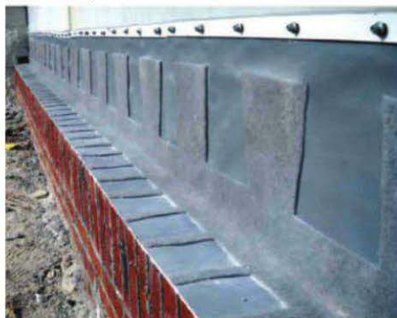
Unitized flashing systems can be specified using any of the most common flashing materials.
