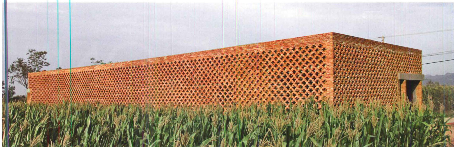
The architect was inspired to design the brick screen after a visit to the westernmost areas of China, including Kashgar in Xinjiang province. The screen helps keep the house cool in summer and warm in winter (above). An angled concrete roof collects and stores rainwater and provides a place to dry food (left and below left). Two women live in the house, which is also used for a women's weaving cooperative (below).
