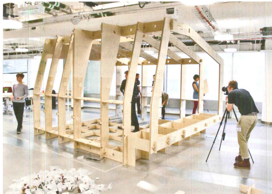
Components of the WikiHouse building system by London-based OOZ/ can be downloaded and "printed" using a CNC milling device and then assembled. The firm has built five prototypes so far, but its goal is to refine the construction process and turn it over to users rather than devise a specific blueprint. Residents can customize the system to fit their housing needs and local context.
