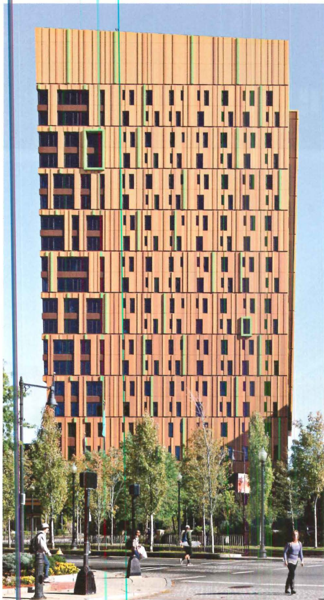
ART PROJECT Over 5,500 composite-metal panels in five custom colors, widths, and depths, combined with energy-efficient windows, make up the facade of MassArt's new residence hall (left and above). Below, a breakdown of the different color panels used in the facade; the colors get progressively lighter toward the top.
