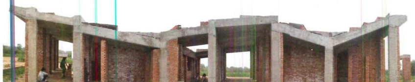
The architect was inspired to design the brick screen after a visit to the westernmost areas of China, including Kashgar in Xinjiang province. The screen helps keep the house cool in summer and warm in winter (above). An angled concrete roof collects and stores rainwater and provides a place to dry food (left and below left). Two women live in the house, which is also used for a women's weaving cooperative (below).
