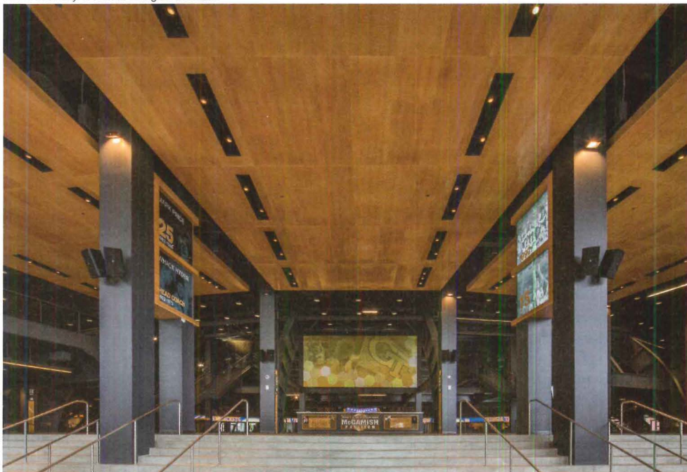
Powder-coated large-format ceiling panels simulate wood at the entry area for the new Georgia Tech arena designed by Populous. The panels conform to the ASTM E-84 Class A fire rating required by code and required less time to install than heavier composite wood panels.
