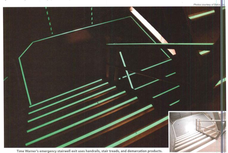
hotoluminescent (PL) technology saves lives by lighting a glowing path for a critical duration of time to evacuate occupants and navigate stairways during extreme circumstances like total darkness due to loss of power in a multistory building. PL glows through darkness and smoke-filled stairways, allowing first responders to get in and find their way to alleviate the threat and evacuate building occupants in a manner that is safer for everyone.
