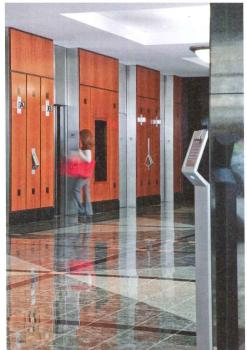
Computer-based elevator destination control systems allow users to indicate their destination before entering the car.
