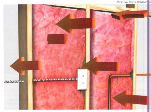
Traditional fibrous batt insulation is prone to incomplete filling of the stud space cavities, allowing greater heat transfer than desired.
