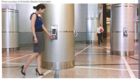
The addition of access-card readers to the user control panel allows customized service.
