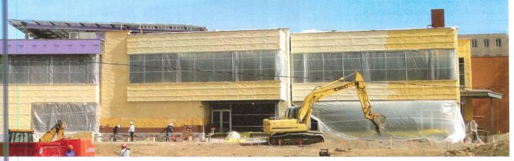
Me lium-density closed cell insulation can be spray applied to the outside of the sheathing on a stud cavity wall assembly and remain durable and water resistant during the construction period.
