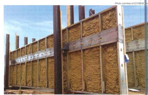
Low-density open cell spray foam insulation has been installed to fill and seal stud cavities of this prefabricated wall panel and shipped to the site for final installation.
