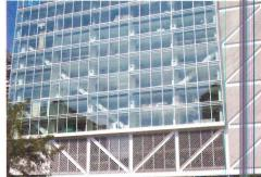
To accomplish the building's engineering feat, the entire building was designed as a truss with the structure incorporated as an exposed design element.
