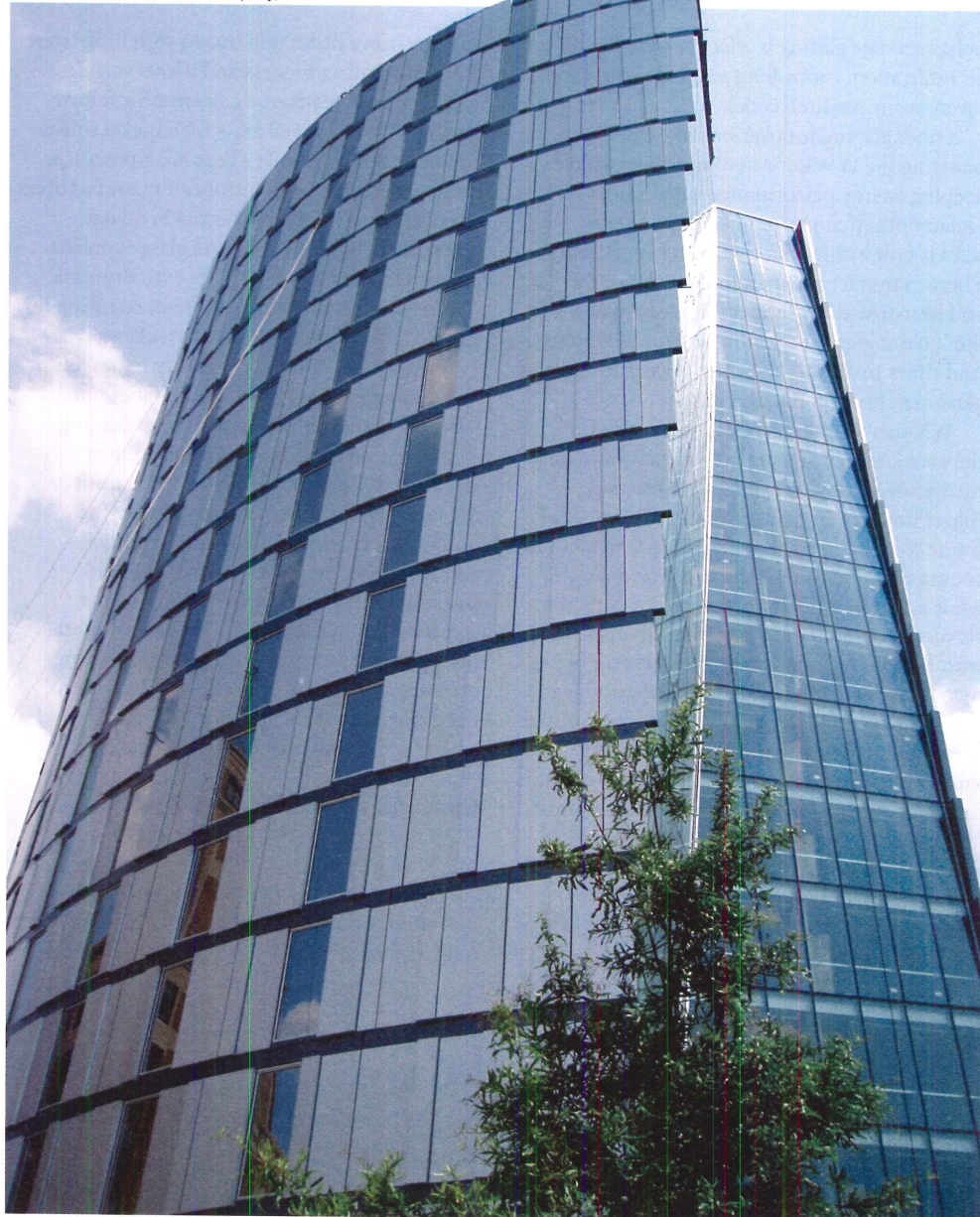
At Drexel University, the new Millennium Residence Hall features a unitized curtain wall that was specified to have coordinated glass panels and aluminum composite panels, all provided by the same manufacturer.
