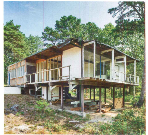
The Weidlinger house, shown here during reconstruction.
