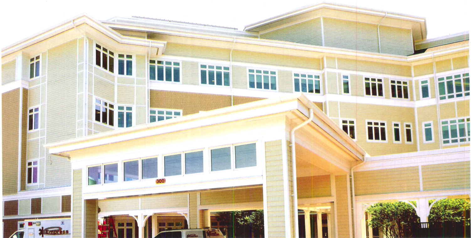
For the LEED-certified Elizabeth Seton Pediatric Center, a long-term-care facility for 130 children in Yonkers, New York, the firm Perkins Eastman specified crisp, white vinyl frames for new picture windows and casements using low-E glass with argon gas fill.
