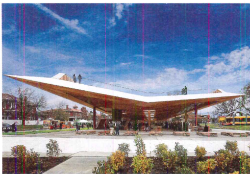
G8WAY DC Category: Custom Solutions Location: Washington, DC, USA Architect: Davis Brody Bond Engineer of Record: Robert Silman Associates Precast Producer: Gate Precast Company Photo: Eric Taylor, Davis Brody Bond
