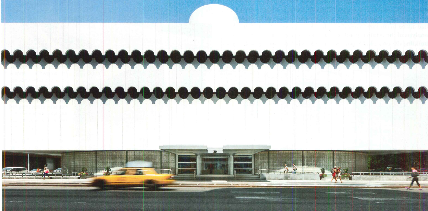
Perkins Eastman restored Albert Ledner's 1964 National Maritime Union headquarters in Manhattan's West Village, and inserted a stand-alone emergency department inside.
