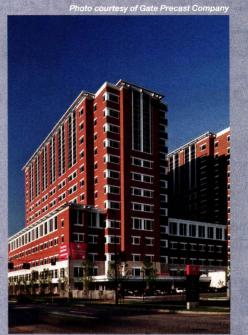
The precast included several different finishes with five colors of thin brick, producing a range of color that is common to the handset-brick and stone used on adjoining buildings.
