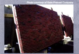
Precast panels consist of a 3-inch exterior wythe of concrete, with a 5/8-inch layer of embedded thin brick, a middle 2 inches of insulation with ship-lapped edges, and an interior 4-inch structural wythe. Thin brick can also be returned for edges and corners if desired as seen in this photo.
