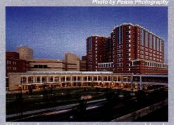
High-performance precast concrete combined a continuous air and vapor barrier, as well as continuous insulation, efficiently into one system. This provided a calculated performance R-value of R-26.
