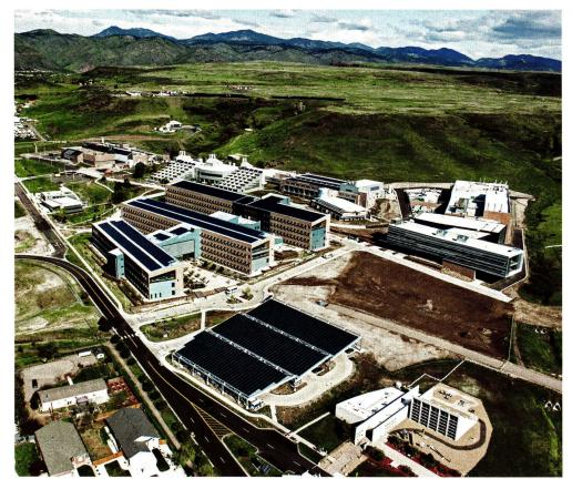
**RESEARCH SUPPORT FACILITY** An office building on the Golden, Colorado, campus of the National Renewable Energy Laboratory comprising three wings (left) relies on a number of tightly coordinated strategies to achieve net zero, including narrow floor plates to facilitate penetration of daylight, and insulated precast cladding chosen for its ability to increase the steel structure's thermal mass.
