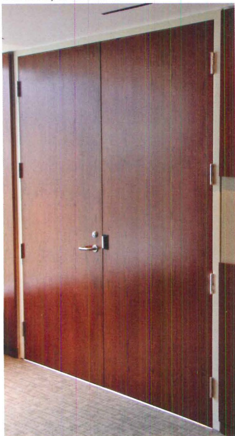
Specialized door, frame, and window systems can be specified to meet performance standards and still feature aesthetic qualities, such as this acoustic wood door and steel frame system achieving an STC rating of 51.
