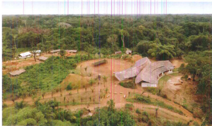
MASS Design Group staked out two circles at the site and placed the curving arcs of the school where the circles meet (above). Many of the villagers had never seen such a large or complex structure before the school was built (right).
