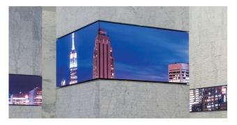
SLICE OF LIFE LED monitors streaming dynamic media are integrated into the marble cladding on the walls and around the columns at the same datum throughout the space (top). These are attached with magnets to simplify removal for maintenance (above).
