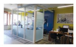
Glass enclosures such as this one can be moved in a quick and inexpensive manner to support changing facility needs and functions.
