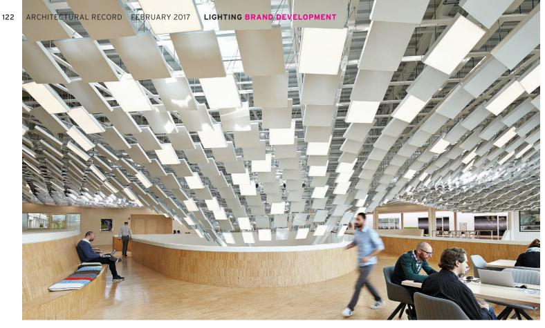
TECHNO COVER-UP Both the light fixtures and unlit panels are made from a Philips ceiling-lighting system that integrates LEDs with sound absorption (above). They are unmodified except for pyramidal reflectors on the reverse side (right). Daylight from skylights (below) is filtered and reflected by the fixtures.
