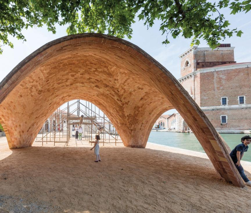
dorf explains. The digital modeling tool they used is similar in concept to the famous experiments in which the Spanish architect Antonio Gaudí suspended chains to find the most efficient shape for arches and domes. When slung between two points, a string or chain will inflect to a curve, or catenary, that is uniformly loaded in tension. If that shape is inverted and constructed of a rigid material like masonry, it forms an efficient arch in compression.
