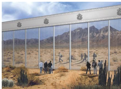
Penna Design of Fort Worth submitted two proposals, one of which consists of steel columns and double wire mesh to allow for visibility. The design calls for the incorporation of the U.S. seal as well as "neoclassical architecture influences."
