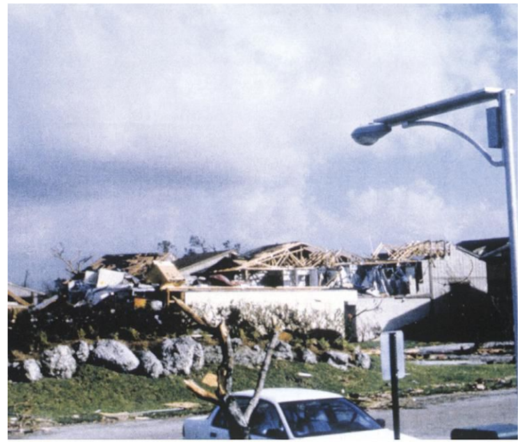
Photos courtesy of the National Renewable Energy Laboratory/Solar Outdoor Lighting
