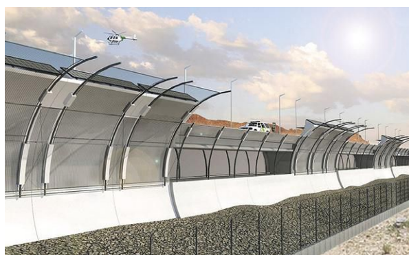
Collaborative Design Architects in Billings, MT, was inspired by concave hydroelectric dams in the area to build a "better barrier." The multipurpose concept features photovoltaics and a roadway for border-patrol vehicles. Its hollow core could house resource pipelines.
