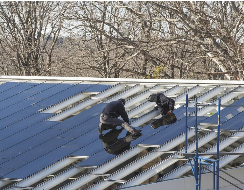
INSTALLATION OF NEW CUSTOM GLASS PANELS AT PHILIP JOHNSON'S SCULPTURE GALLERY
