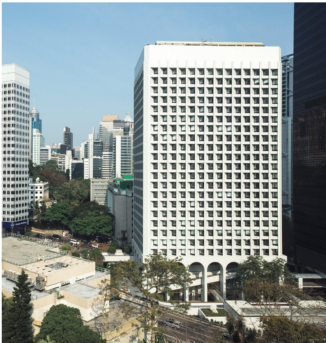
THE HIGH ROAD The Murray Hotel occupies the 1969 Murray Building, where a former parking lot deck has been opened up to reveal a new plaza (opposite), with a 120-year-old cotton tree. Built for government offices, the concrete structure is on a prominent sloping site in Hong Kong's Central district (above).
