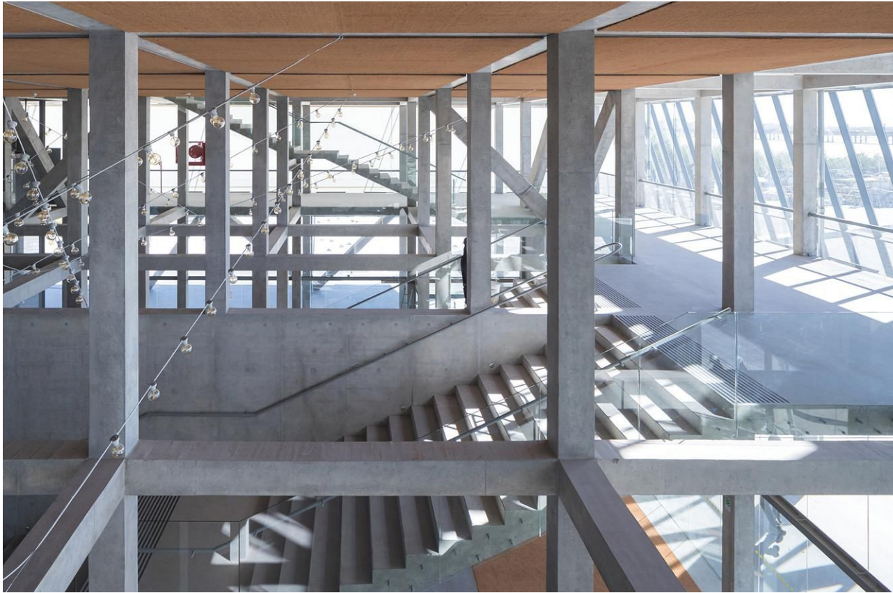
JUNGLE GYM The interior is a grid of slender concrete columns and beams, intersecting with straight and spiral stairs (left and opposite); the main theater (below).
