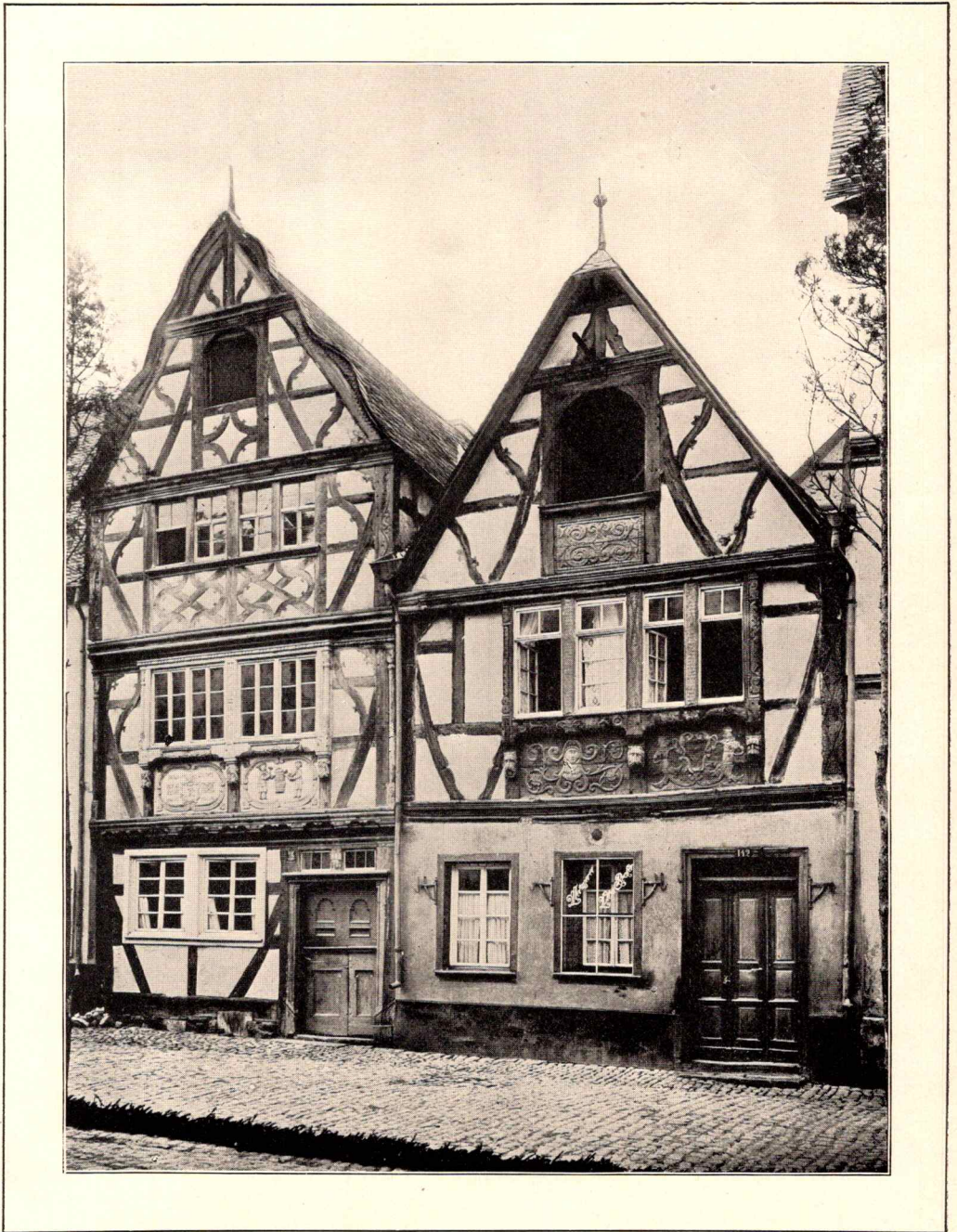
HOUSES IN RHENSE (1671 AND 1652)
