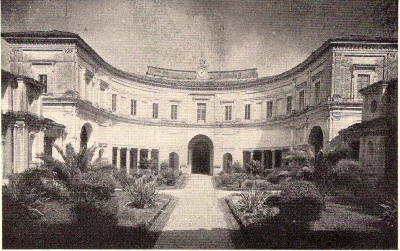
VILLA PAPA GIULIO, CASINO, COURT FAÇADE
