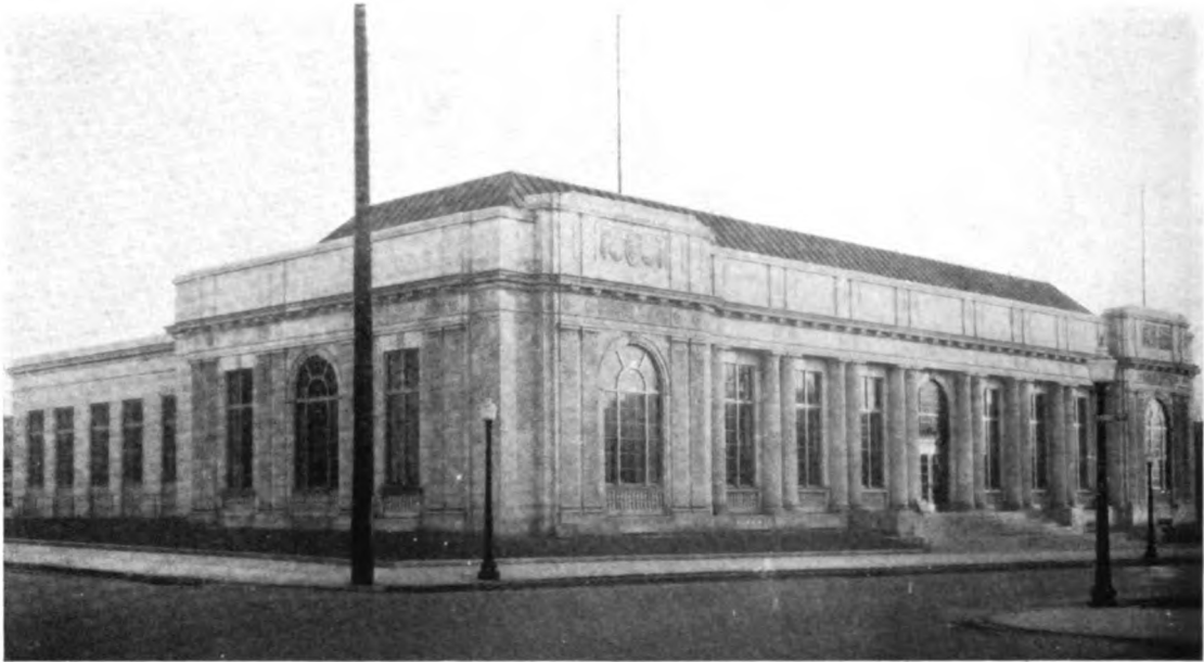
UNITED STATES POST OFFICE, LIMA, OHIO Built of Variegated Limestone from B. G. Hoadley Quarries, Inc., Cut by The Edward Edinger Company.
