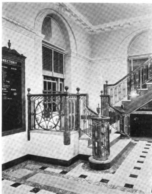
Interesting bronze treatment of stairway in lobby of Post Office at Lowell, Mass.
