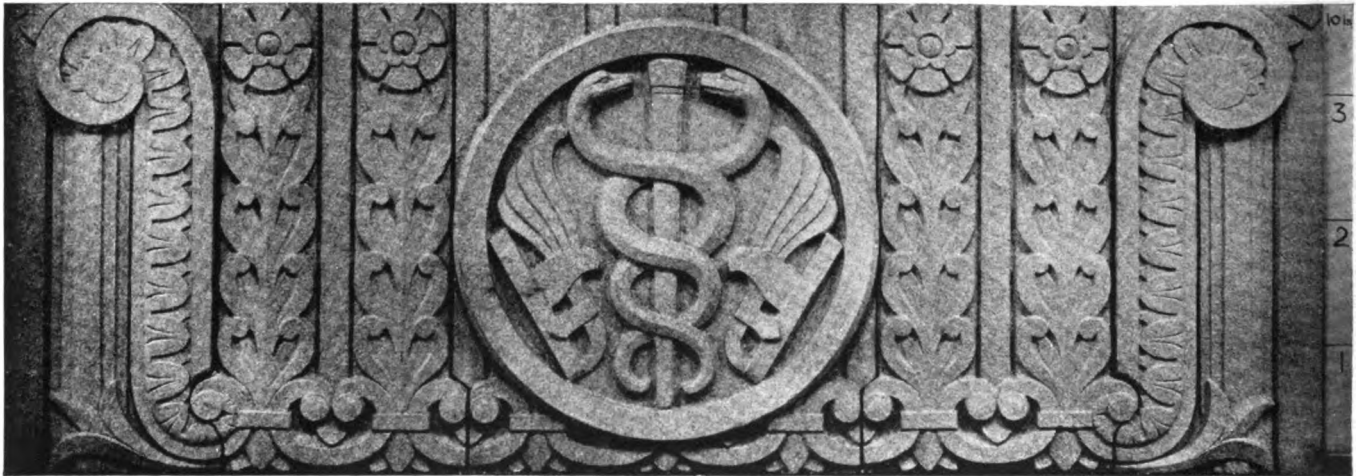
Detail of terra cotta granite spandrel panel. Note jointing scale.
