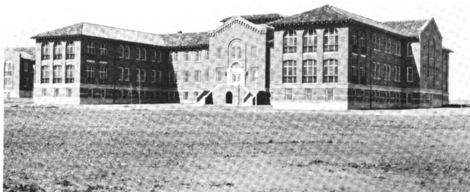
CONTINUED TREATMENT BUILDING, VETERANS' ADMINISTRATION HOSPITAL, WACO, TEXAS
