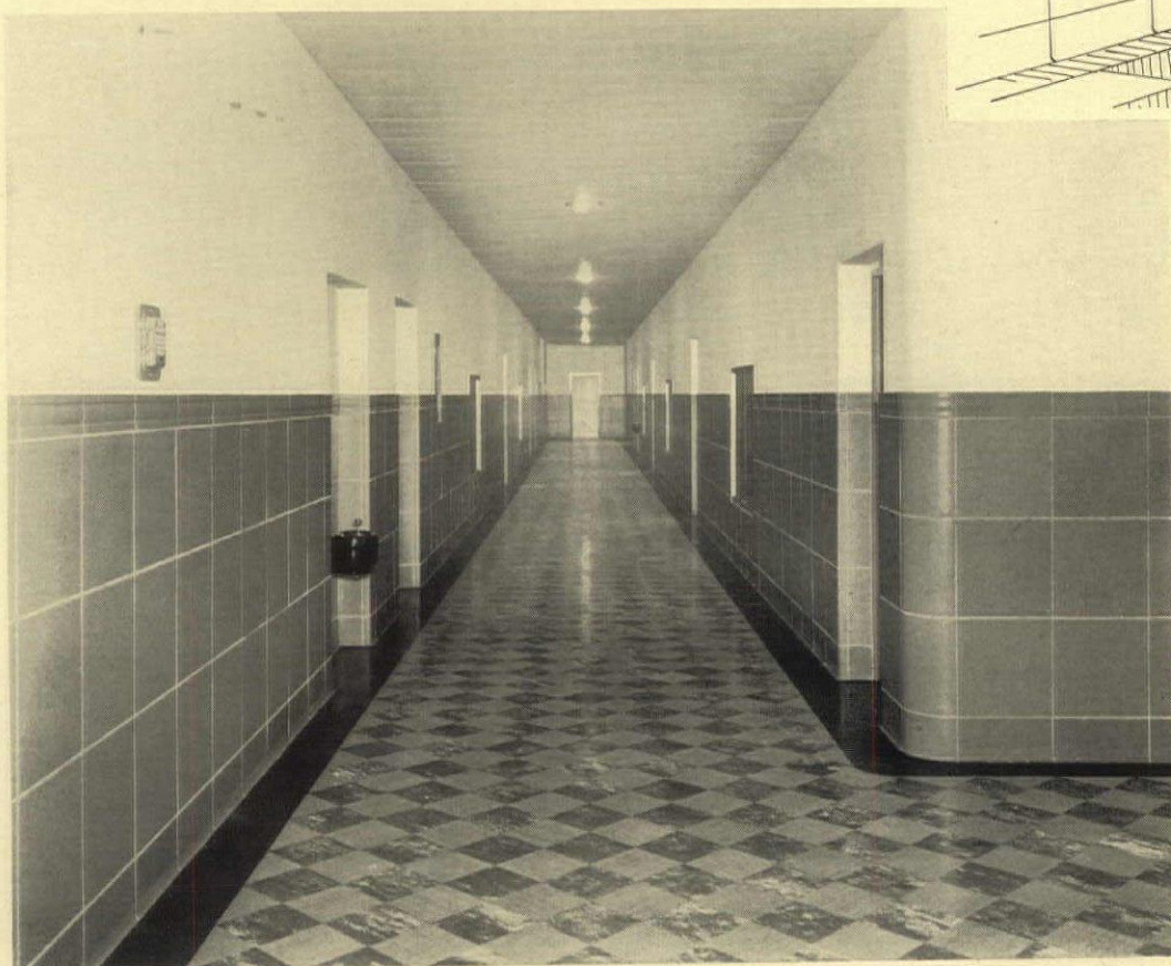
Terra Cotta Wainscot, Unit size 16" x 16", School, East Northport, N. Y. J. Van Alst, Architect.
