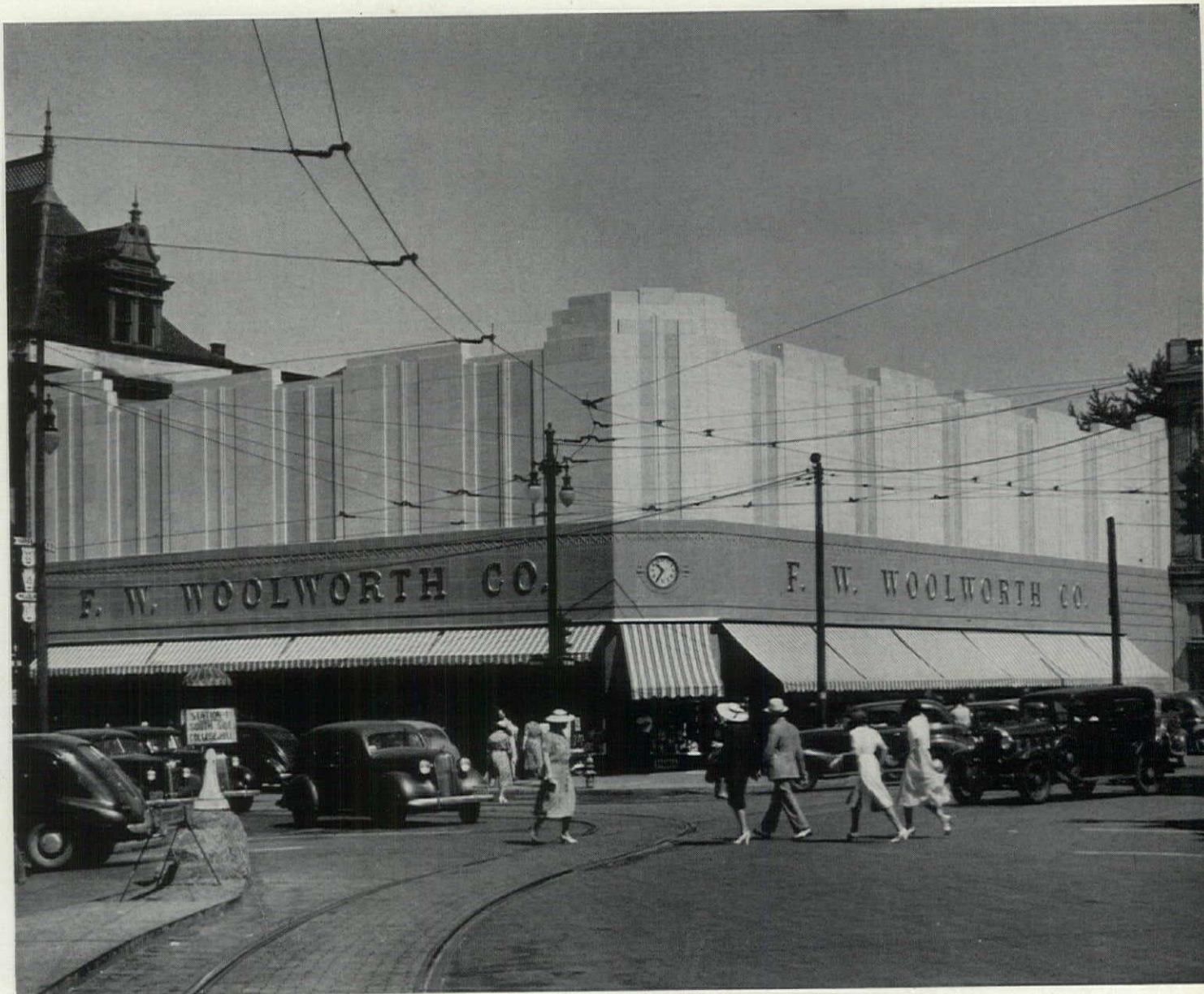
STORE FOR F. W. WOOLWORTH CO., EASTON, PA.
